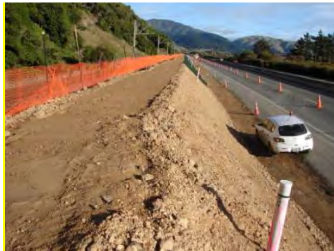
Illustration 10: Preloading adjacent to State Highway
