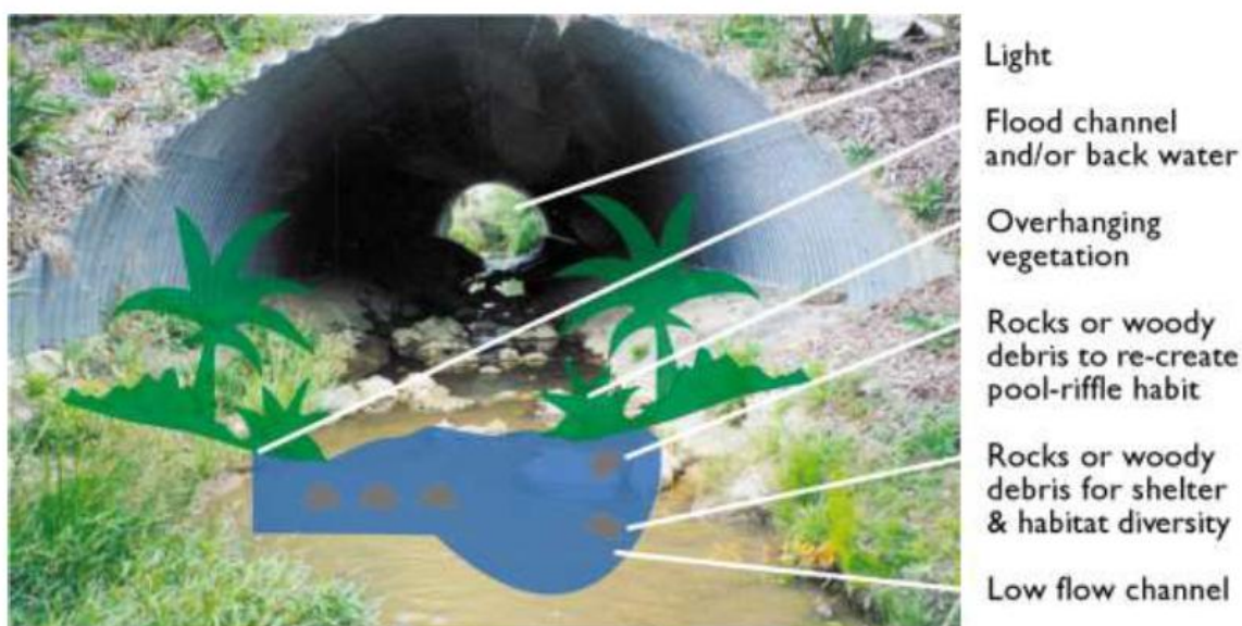
Figure 5 - Example of good fish passage (in a bottomless culvert)
