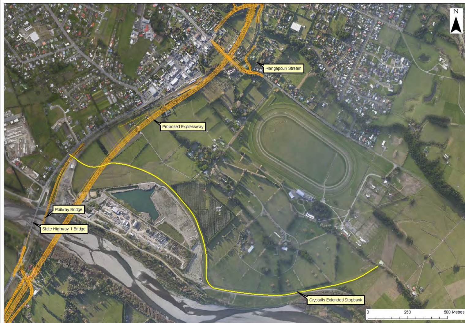
Figure 6.1 Aerial view of Otaki River and floodplain in vicinity of existing and proposed river crossings
