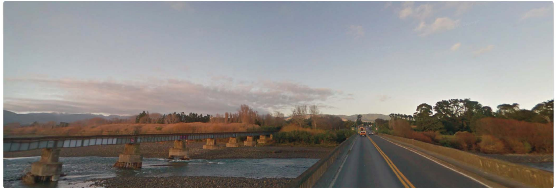
Figure 08. Current SH1 looking south at Ōtaki railway bridge
