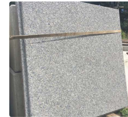
Abutment RE Wall Panels
