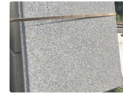
Abutment RE Wall Panels
