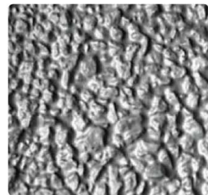
Illustrative - exposed aggregate textured appearance, achieved with a formliner to the triangular face
