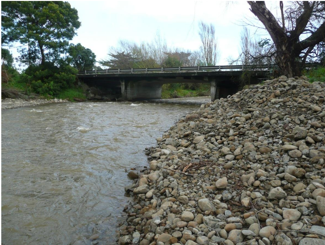
Figure 4-2 Photograph looking downstream at existing State Highway bridge over Waitohu Stream
