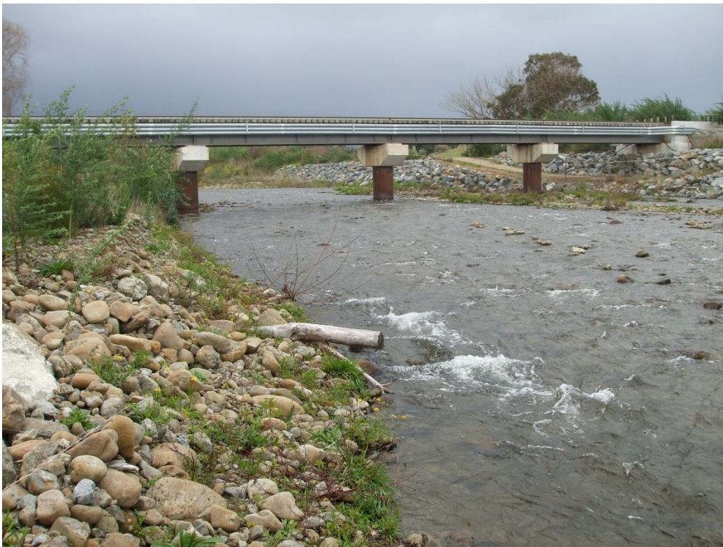
Figure 4-3 Photograph looking upstream at existing NIMT railway bridge over Waitohu Stream
