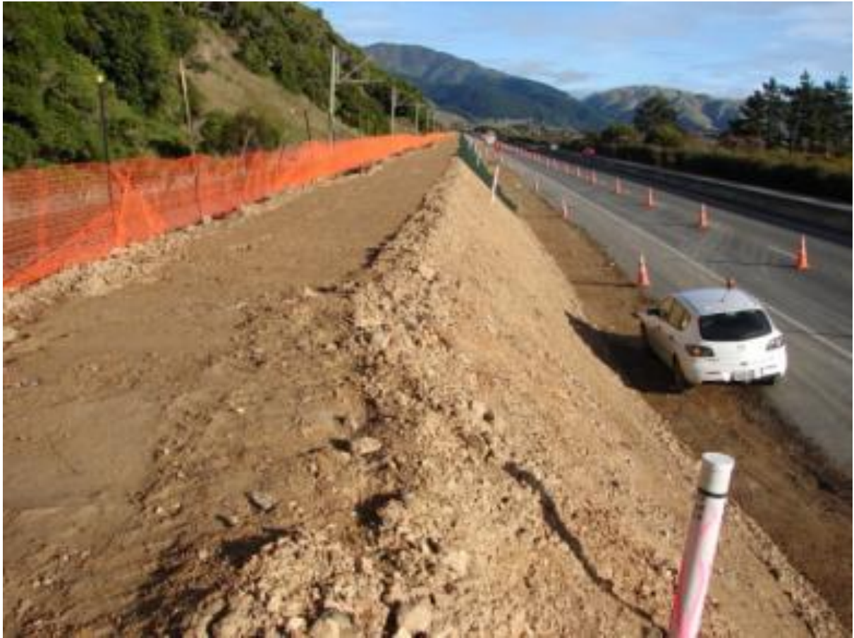
Illustration 16 - Preloading adjacent to State Highway
