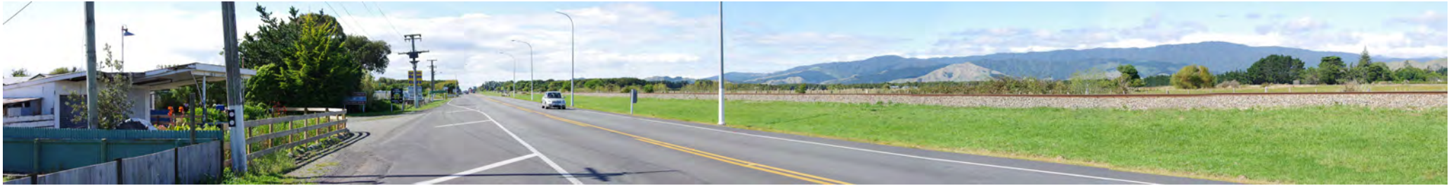
Figure 31. Existing view looking north along the local arterial at Te Horo, towards the proposed Te Horo Underpass
