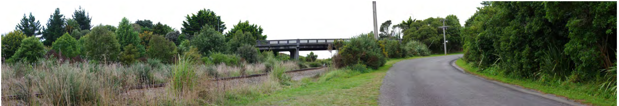
Figure 44. Existing view looking north along County Rd
