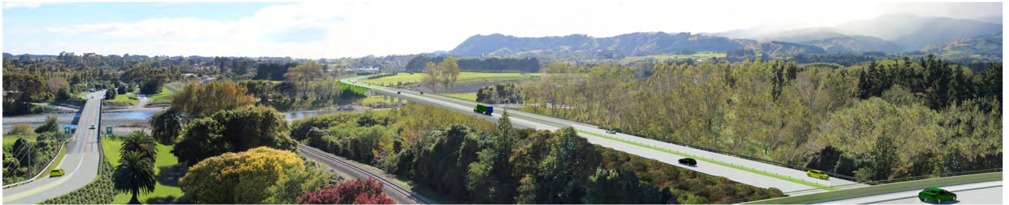
Figure 43. Visualisation of the Project from South Otaki Interchange Refer to Figure 36 for viewpoint location
