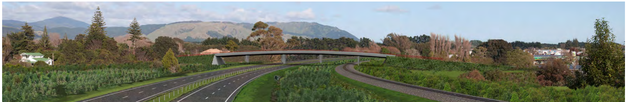
Figure 24. Visualisation looking at the proposed Expressway and Rahui Road Underpass with the proposed Kennedy wetland to the left, and reconfigured Pare-o-Matangi Reserve to the right
