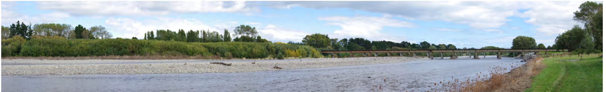
Figure 21. Existing view of the SH1 and NIMT railway bridges from Chrystalls Bend Walkway
