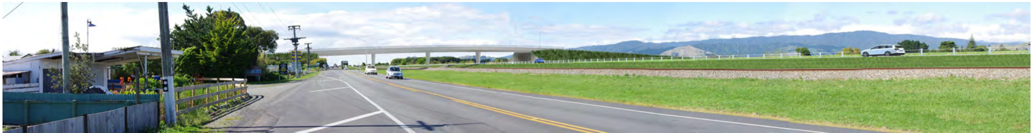
Figure 32. Visualisation looking north along the local arterial at Te Horo, towards the proposed Te Horo Underpass
