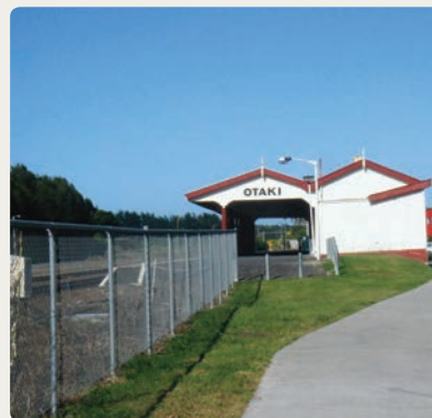
Realignment of Ōtaki Railway Station is proposed as part of the expressway project
