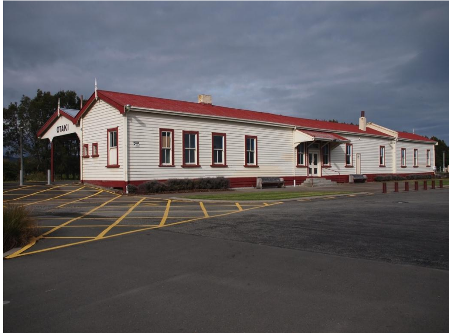
Figure 5 Ōtaki Railway Station, photo I. Bowman, 11 May 2012
