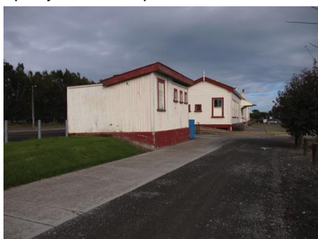
Figure 14 Toilet block to the north of the station, photo I Bowman, 11 May, 2012
