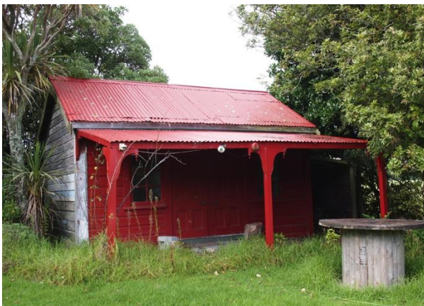
Figure 11 Former (railway?) hut, photo I Bowman, 11 May, 2012
