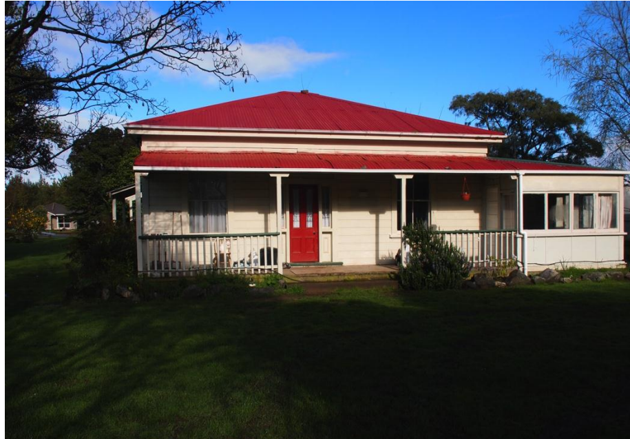
Figure 14 'Clifden' at Bridge Lodge, photo I. Bowman, 11 May 2012
