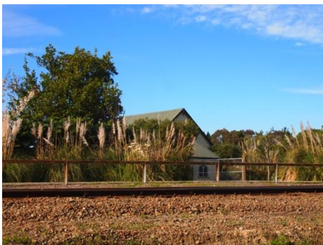
Figure 20 setting to the west of the former Rahui Social Club building, photo I Bowman, 11 May, 2012
