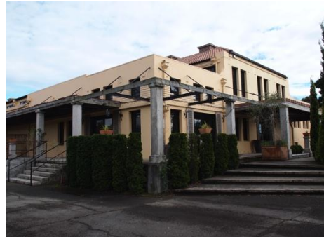
Figure 17 refurbished Milk Treatment Station with planting, photo I Bowman, 11 May, 2012
