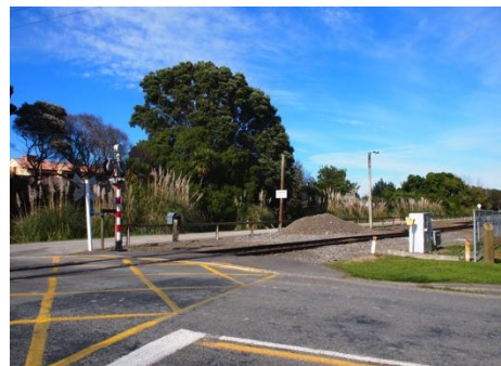
Figure 19 view from the corner of Country Road and Rahui Road with the railway line in the foreground, photo I Bowman, 11 May, 2012
