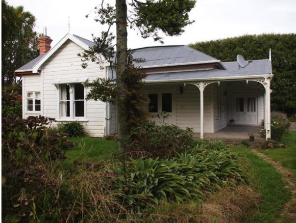
Figure 13 house formerly owned by Mirek Smíšek, photo I Bowman, 11 May, 2012
