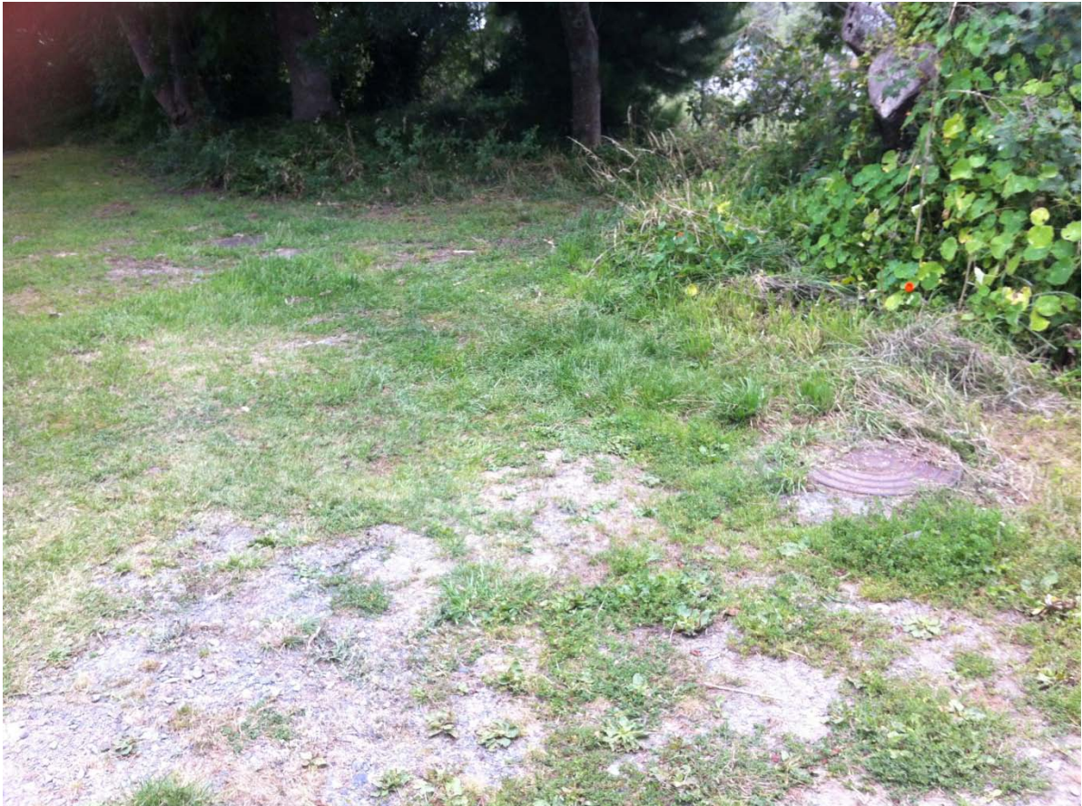
Photograph 5: Western septic tank
