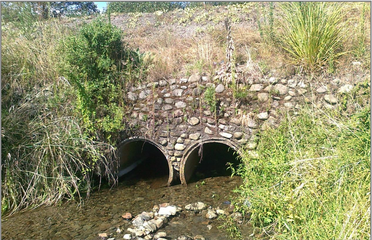
Photo of existing outlet
