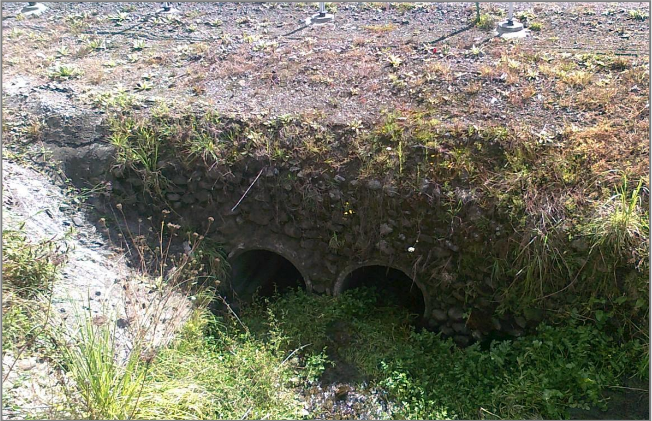
Photo of existing inlet
