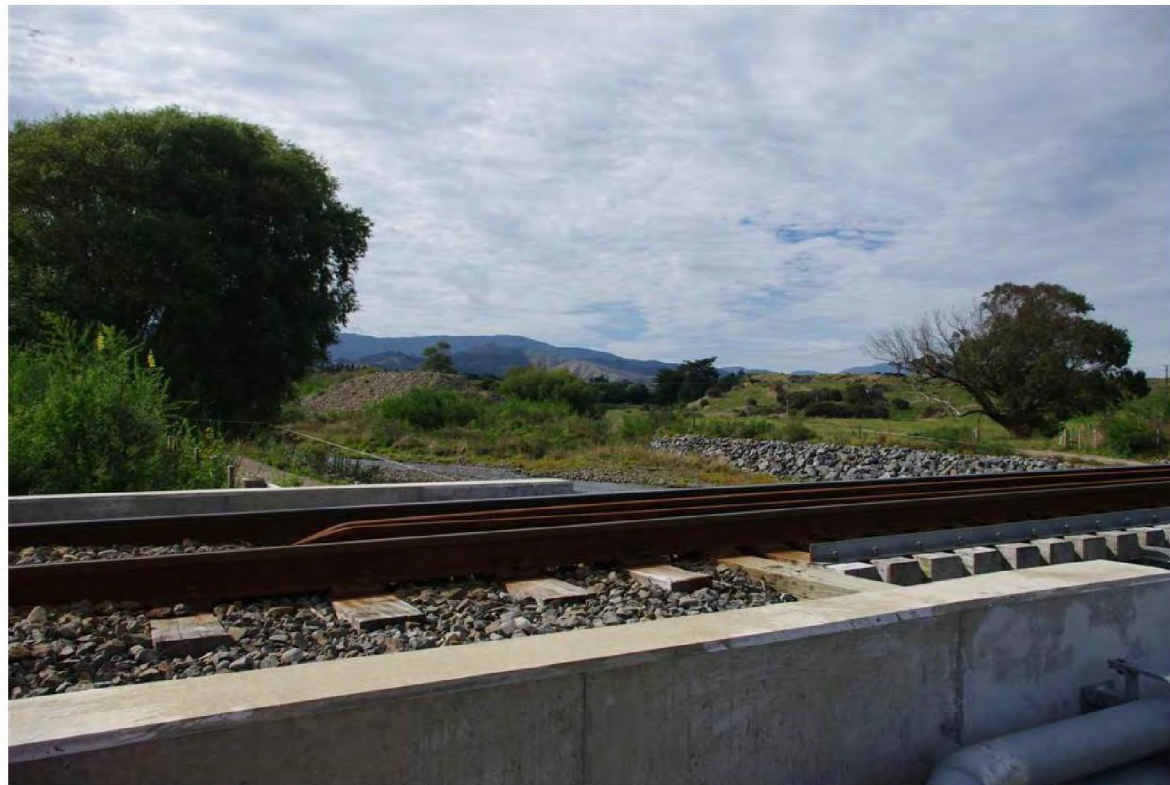
Photo 2: Taylors Rd to Waitohu Valley Rd – NIMT Railway/Waitohu Stream Bridge (Looking east and upstream – Expressway will traverse from behind gravel stockpile in middle left across flat paddock in right of photo)
