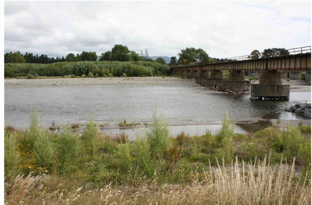
Photo 18: Otaki River – NIMT railway bridge upstream (Looking south – Expressway will cross river on left aspect of photo and transverse through vegetation on south bank)
