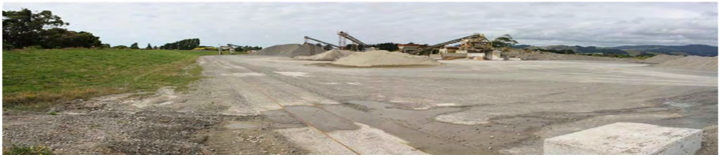
Photo 15: Waerenga Rd to Ōtaki River – Winstone Aggregate area (Looking north – Expressway will traverse across the land immediately beyond the screening plant)
