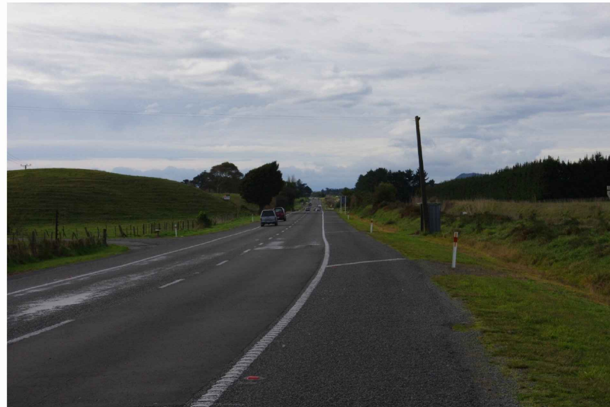
Photo 27: South of Gear Rd to north of Te Hapua Rd – Mary Crest corner north (Looking north – south end of Te Horo straight; Expressway will be on east side of NIMT railway)
