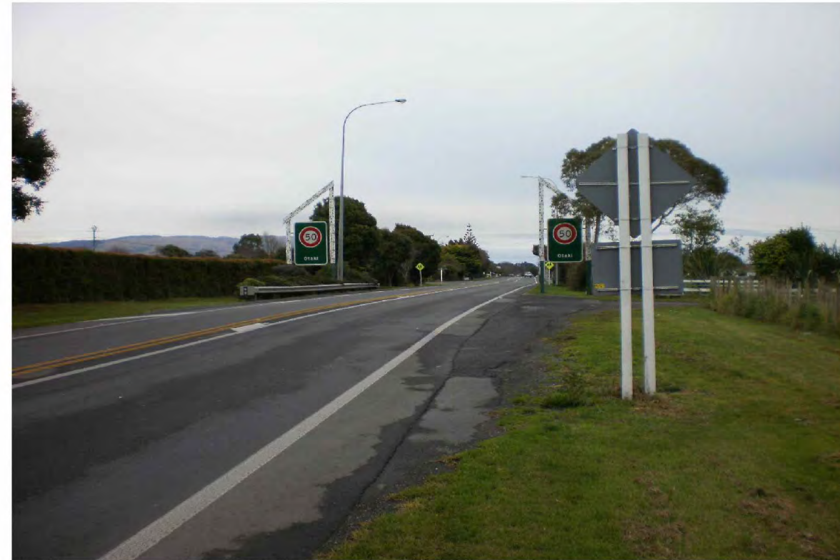
Photo 3: Taylors Rd to Waitohu Valley Rd – existing northern 'gateway' to Ōtaki (Looking south to existing northern 'gateway' to Waitohu 'plateau' area of Ōtaki; existing SH1 alignment will form northern off-ramp to Ōtaki Township)
