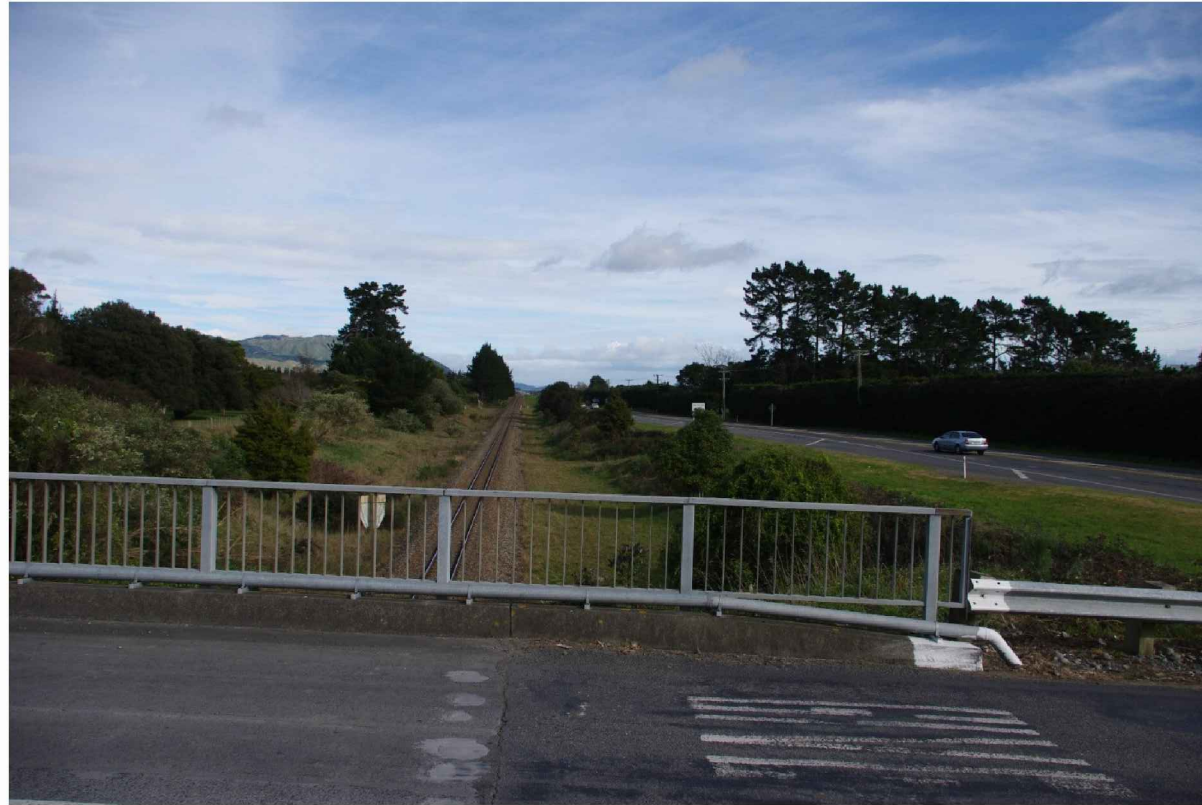
Photo 20: Otaki River to Addington Rd – Otaki Gorge Rd rail overbridge south (Looking south – Expressway will rise from cut to traverse south at grade through centre left of photo)
