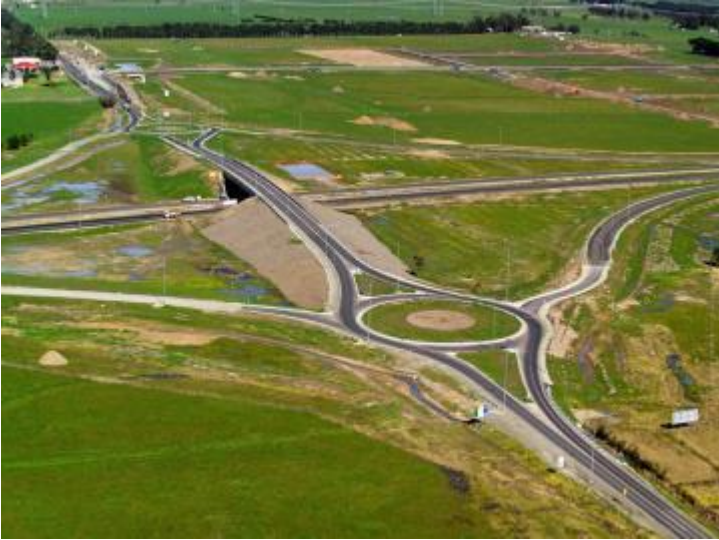
Figure 3 – Service Interchange (Source: AGRD Part 4C)
