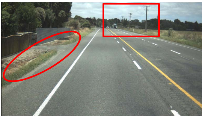
Figure 2-4: Example of SH1 severe roadside hazards (Source: https://www.argonautltd.co.nz/roadrunner/ )
