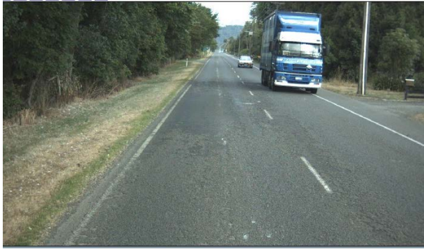
Figure 2-3: Narrow shoulders on SH57 (Source: https://www.argonautltd.co.nz/roadrunner/ )
