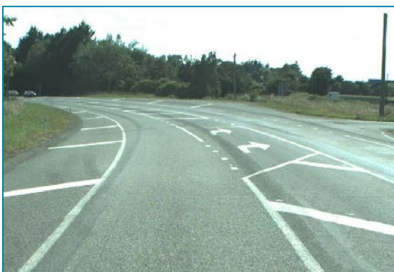
Figure 2-19: Poorly delineated curve and roadside hazards south of Ohau. Old line marking visible
