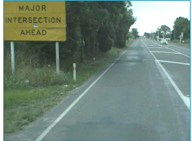
Figure 2-22: Narrow shoulder, trees & old sign north of SH57
