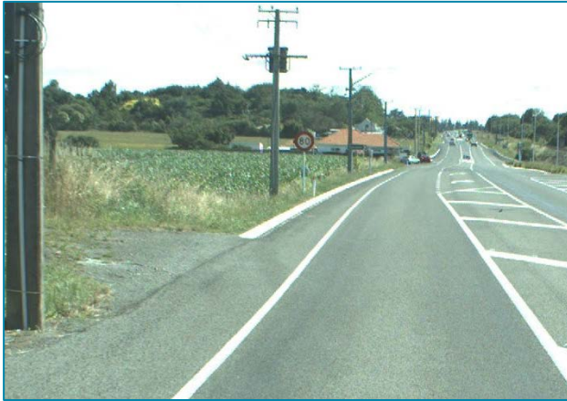
Figure 2-12: Power poles through Manakau Township
