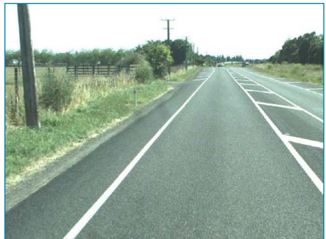
Figure 2-14: Unprotected power poles south of Manakau Rail Overbridge
