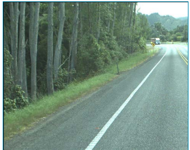
Figure 2-11: Trees and drop-offs south of Pukehou Overbridge
