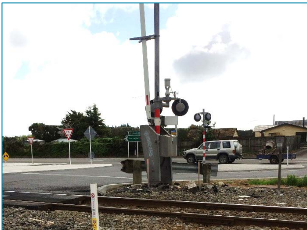
Figure 2-23: Non-compliant safety barrier at SH57 intersection
