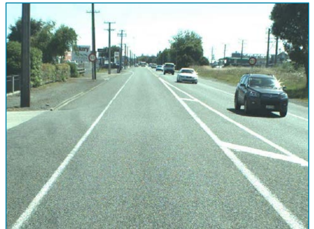
Figure 2-24: Inconspicuous speed limit signs
