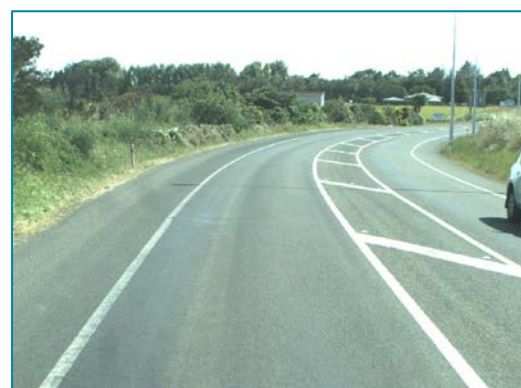
Figure 2-20: Poorly delineated curve and roadside hazards north of Ohau
