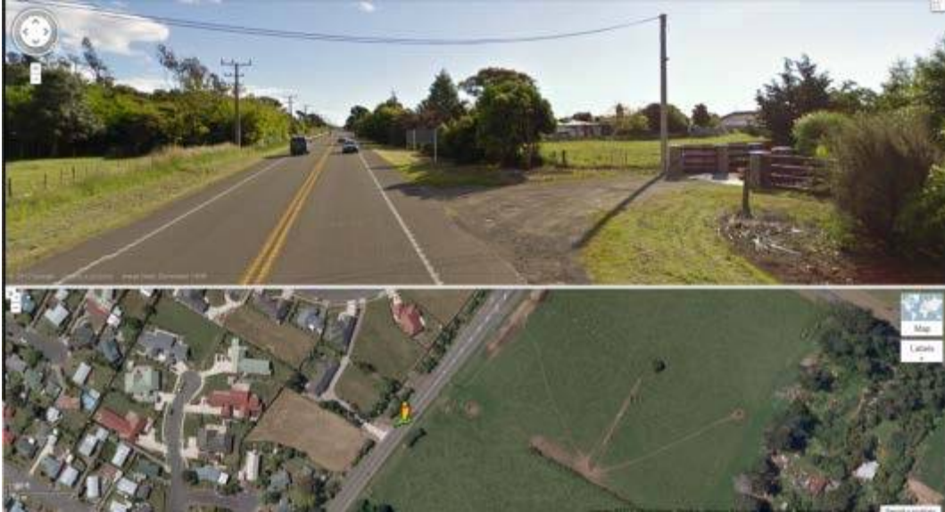
View of the existing accessway approximately 100 m south of the left turn bay into Queen St East
