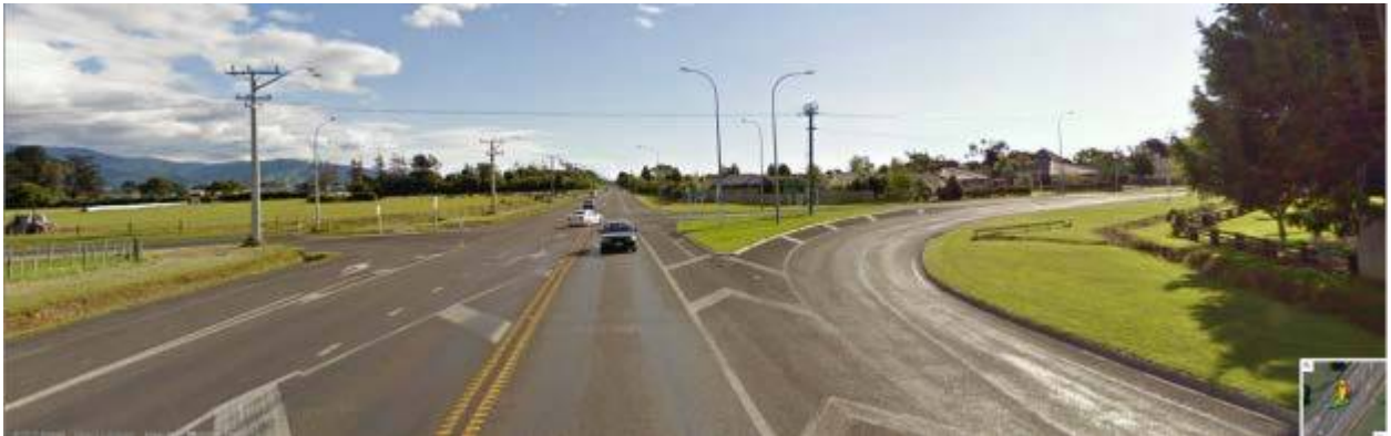
View south-west along SH57
