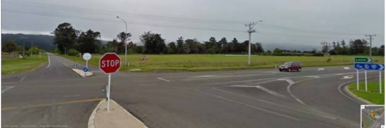
View from Queen St East (Levin approach)
