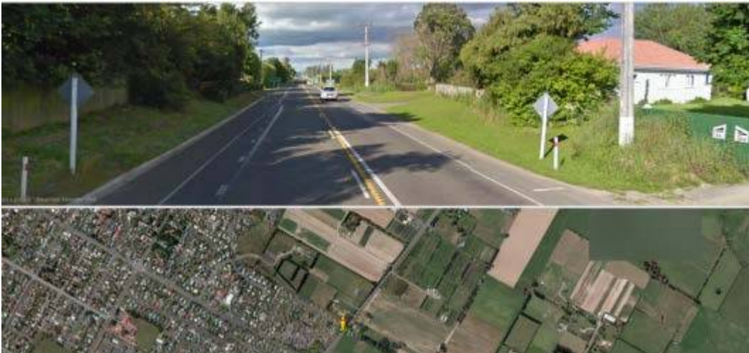
View north-east along SH57 by the end of the acceleration lane from Queen St East
