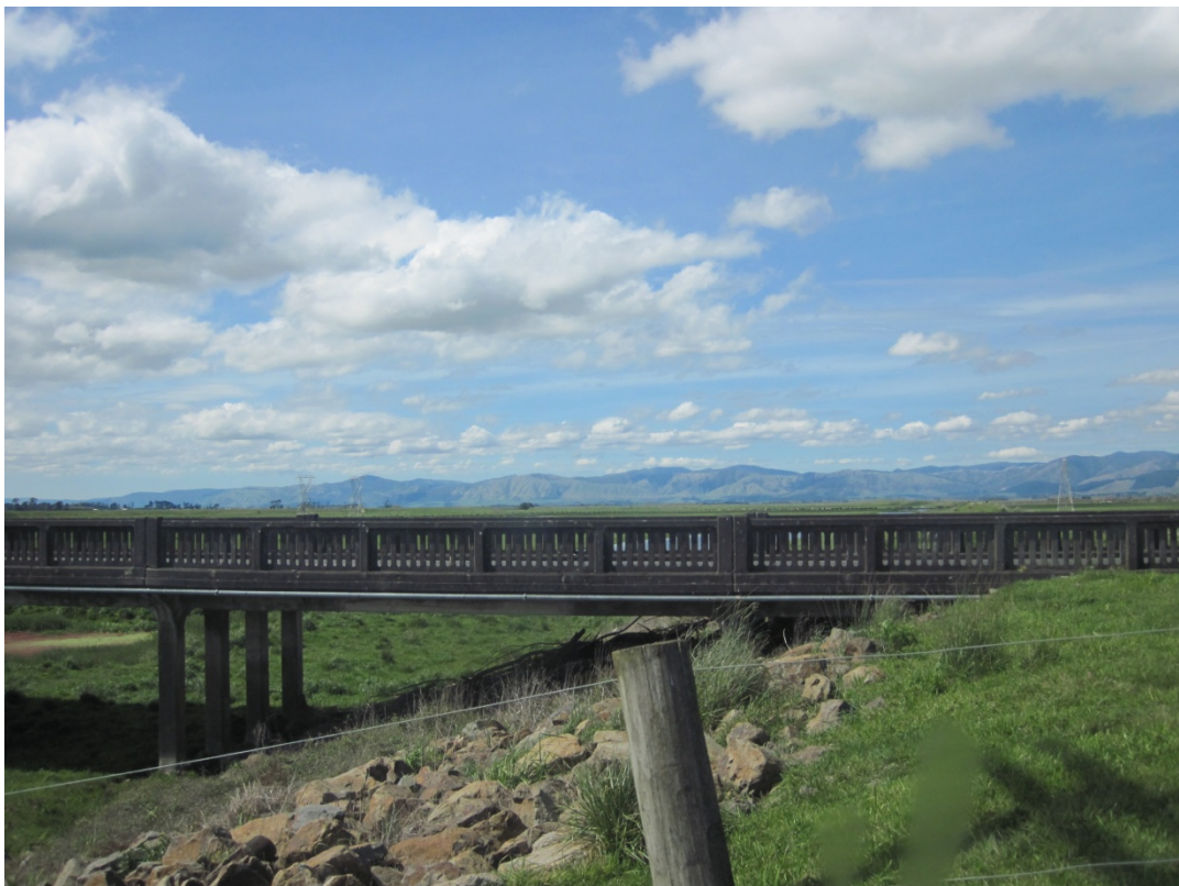
Figure 17-5: Side view of the southern end of the Whirokino Trestle and stopbank
