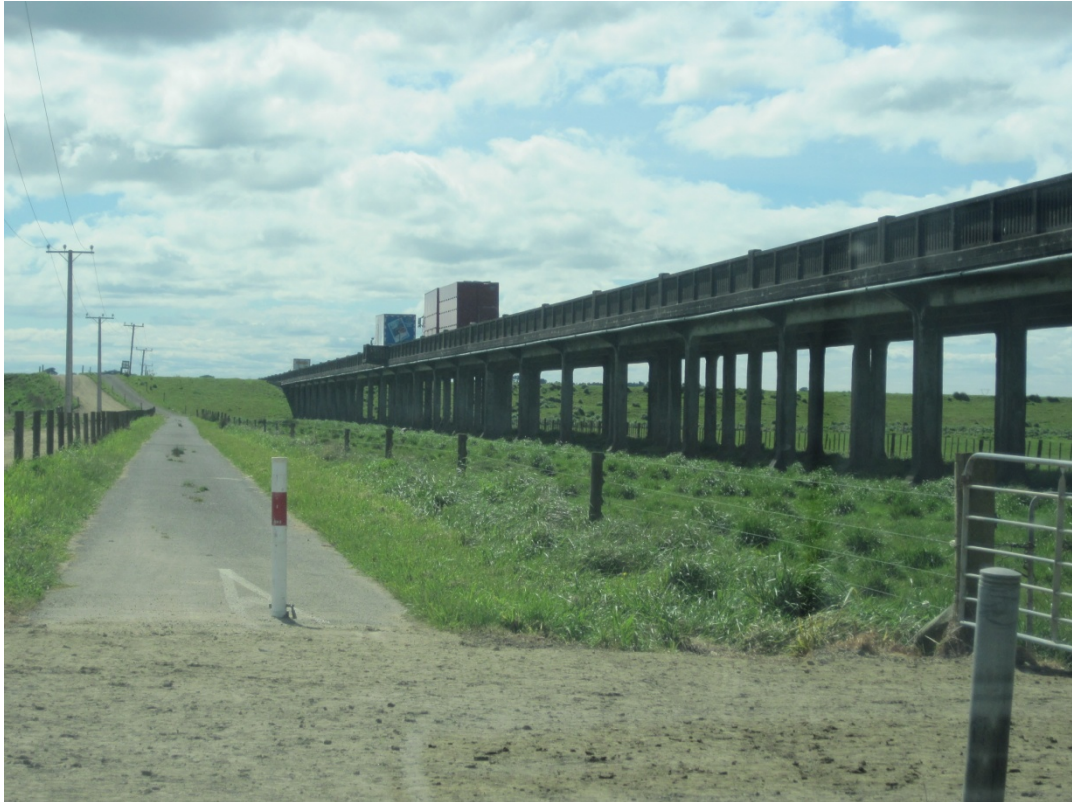
Figure 17-4: View of the Whirokino Trestle from the cycleway (northbound)
