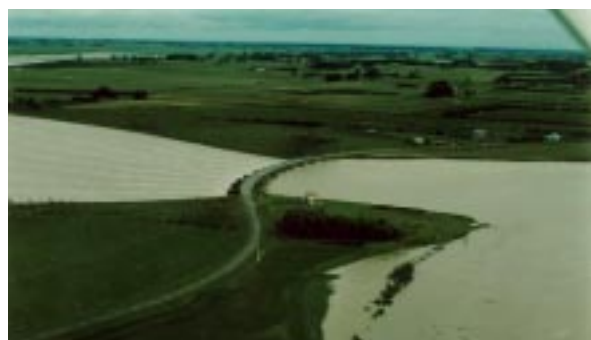
The Moutoa sluice gates in operation
