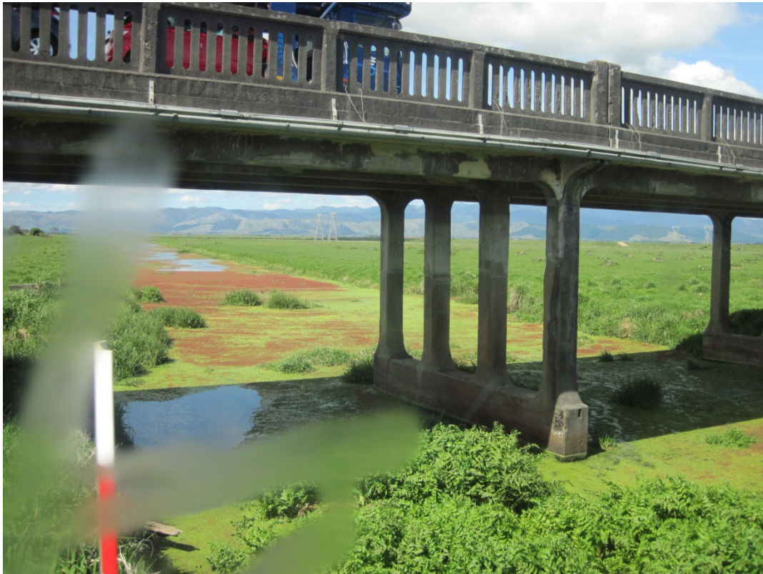
Figure 17-6: Columns of the Whirokino Trestle Underside
