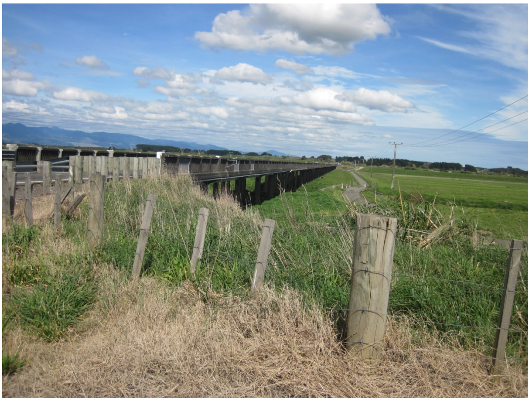
Figure 17-7: View of the Whirokino Trestle and parallel cycleway (southbound)
