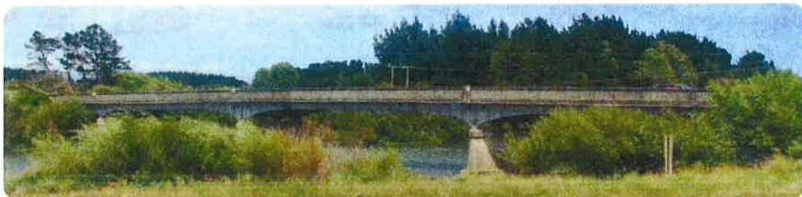
Figure A1.4: Manawatu River (Whirokino) Bridge
