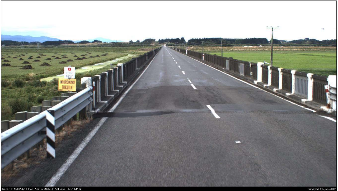
Figure 17-2: Whirokino Trestle Bridge (northbound)
