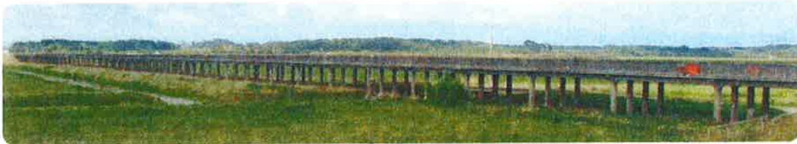
Figure A1.3: Whirokino Trestle Bridge
