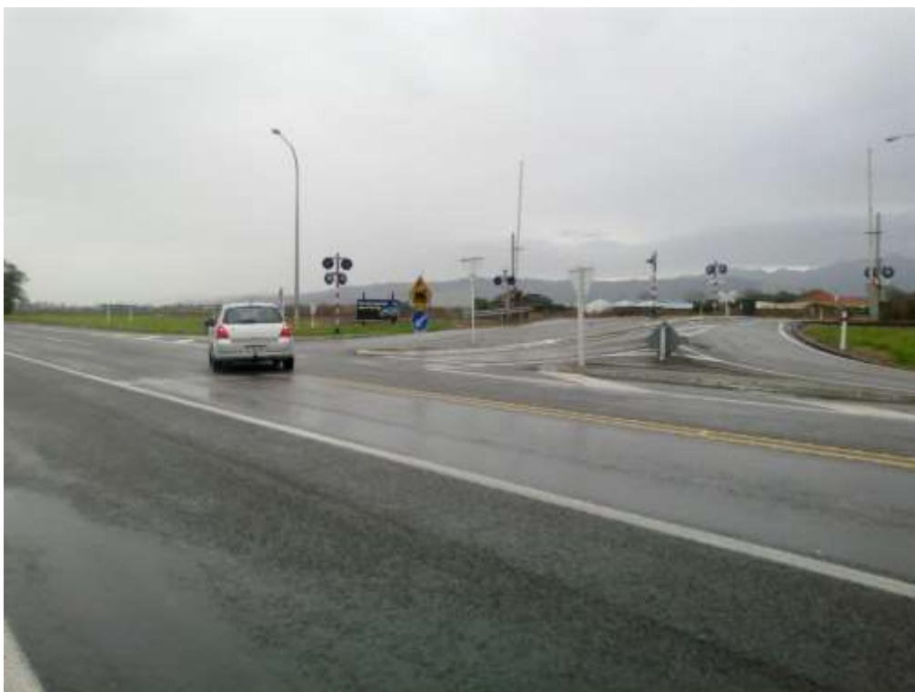
SH1 / SH 57 Intersection
