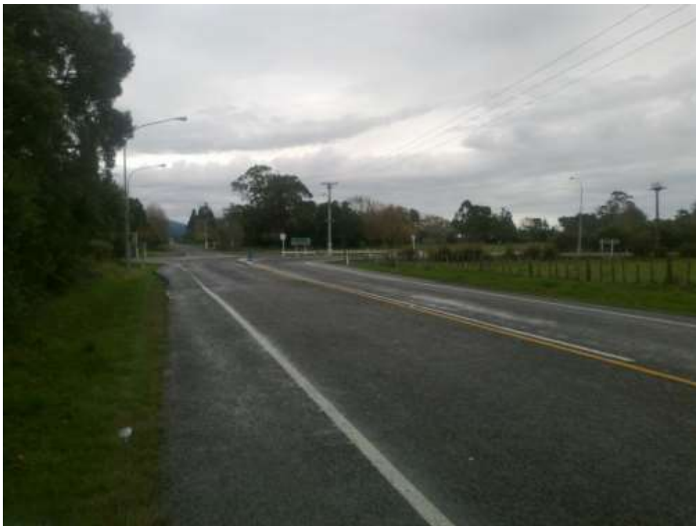
SH57 Arapaepae Road approaching Kimberley Road
