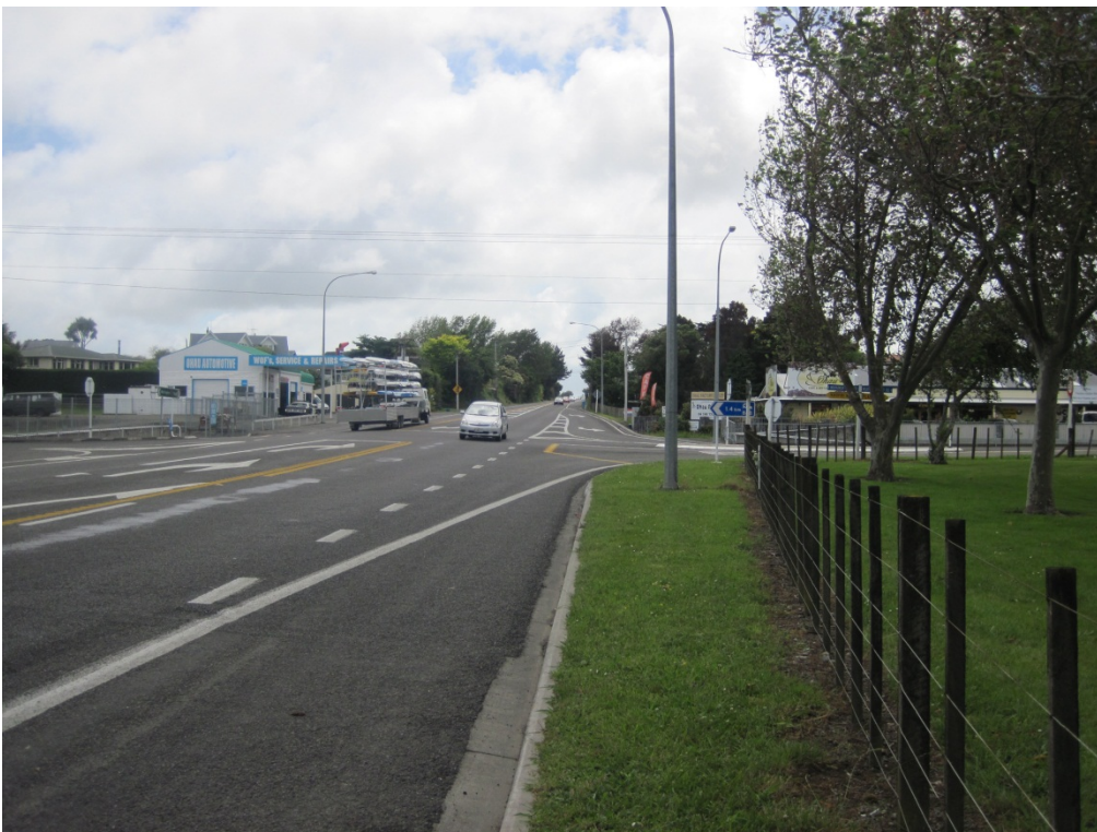
Figure 18-2: Looking north from south of Muhunua Road East
