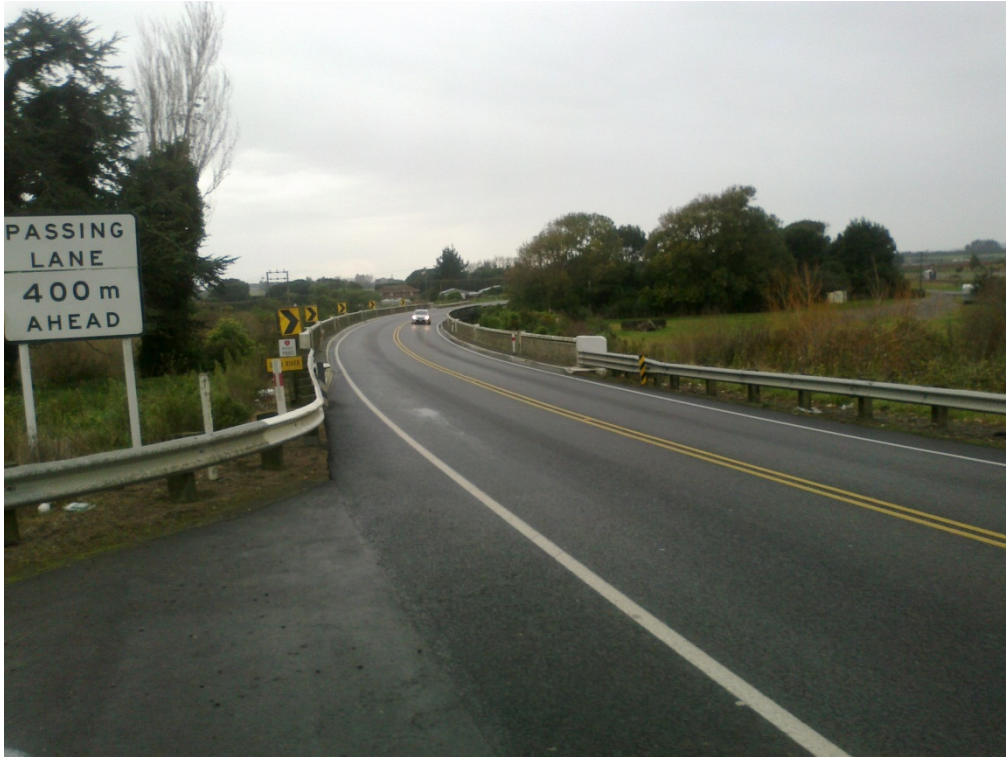
Ohau River Structure Northbound
