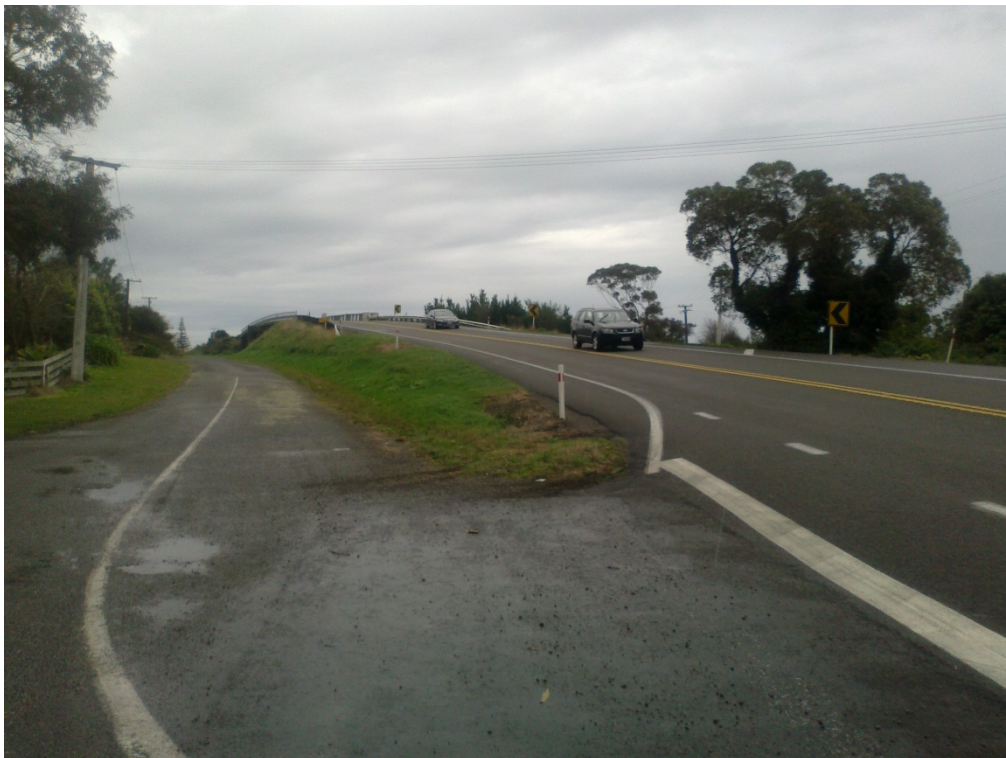
Manakau Rail Bridge Southbound
