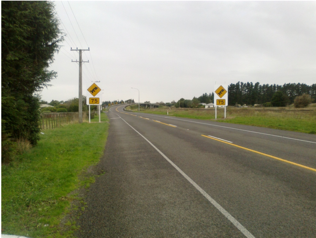
Manakau Rail Bridge Northbound
