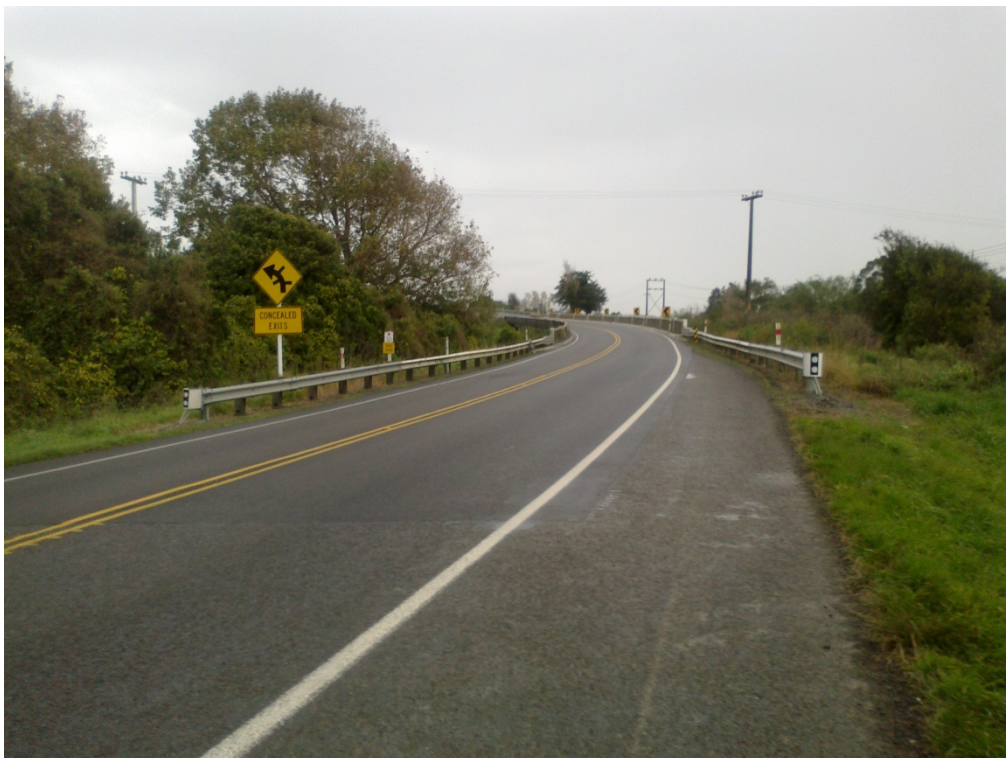
Ohau River Structure Southbound
