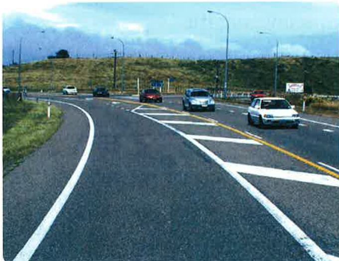
SH1 Walterere Beach intersection
