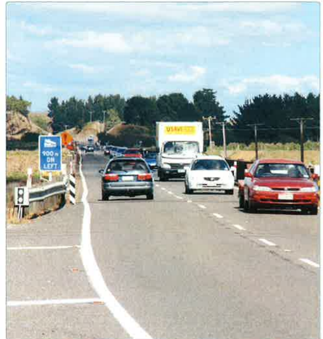
Looking south of Whirokino Trestle, the narrow lanes are evident.
