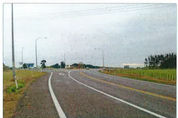
The Waitarere Beach Road intersection as seen when heading north.
