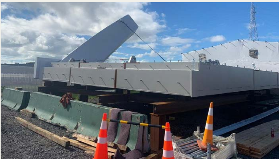
A deck section with the arch was delivered on site
