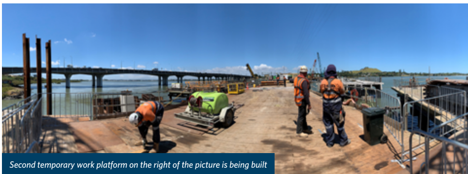
Installation of sheet piles for the cofferdam where pier three will be built
