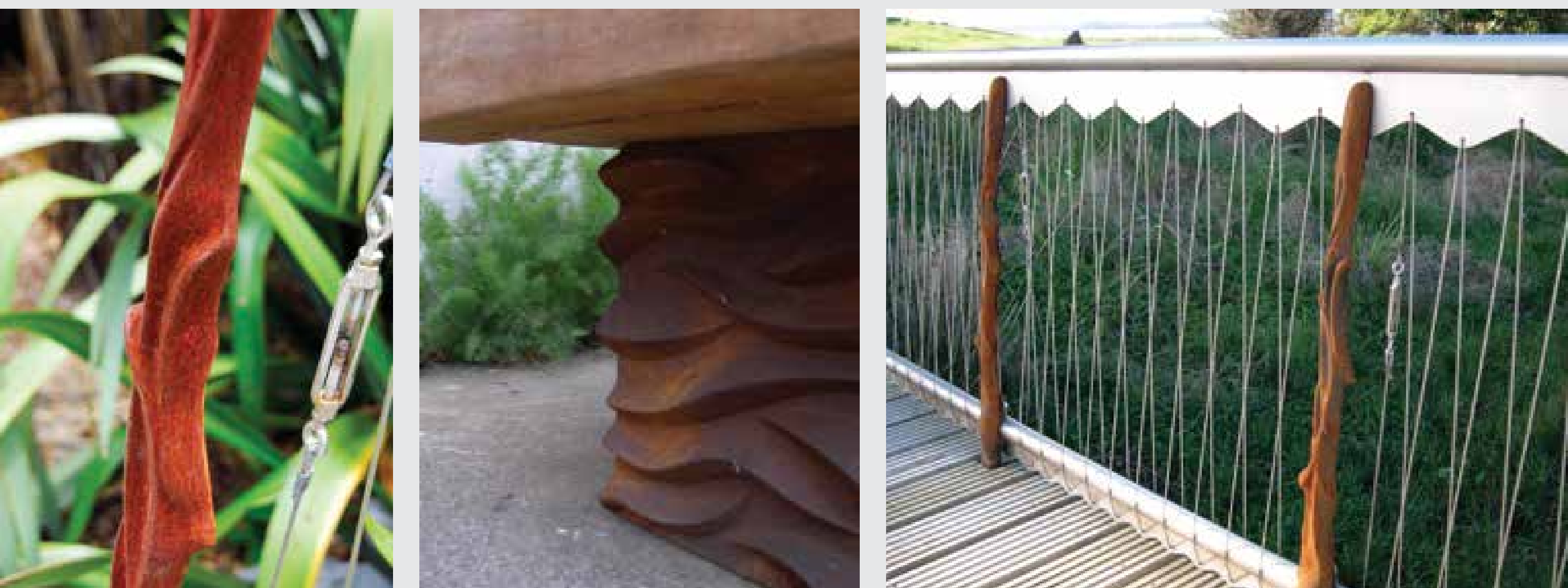
Matthew's work on the Pedestrian Bridges at Orangahina People's Park in Te Atatu
