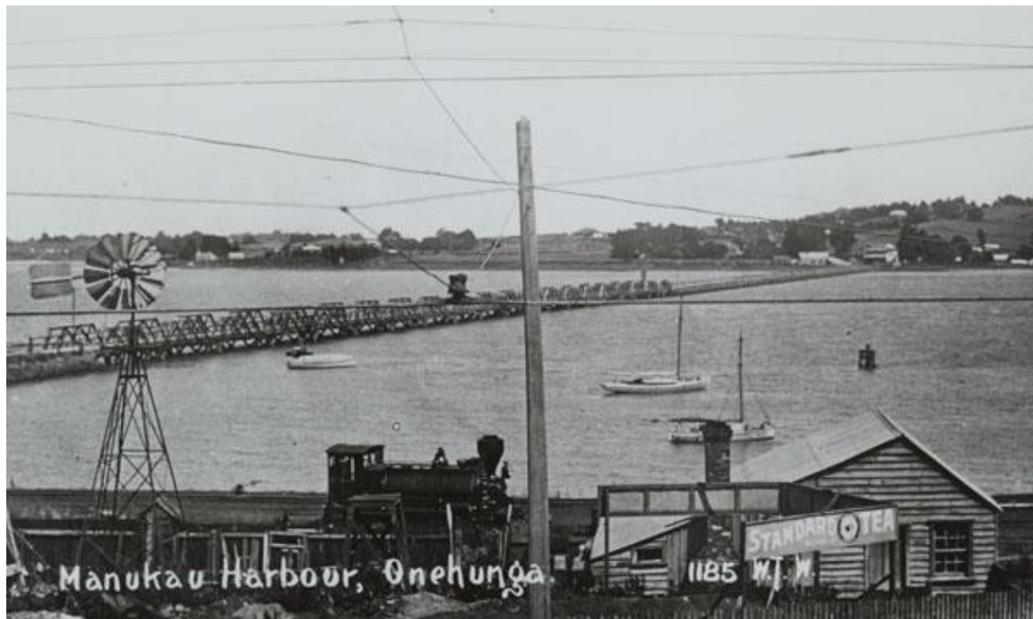
Figure 4: View of the first Māngere Bridge, looking across the harbour from Onehunga, ca 1907. Auckland Libraries Heritage Collections, Footprints 01128, photographer WT Wilson.
