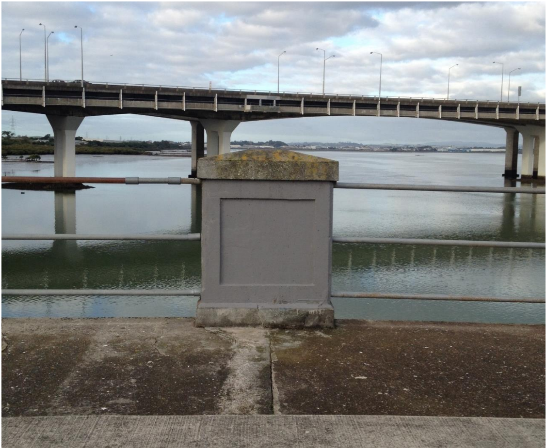
Figure 24: View of a typical concrete pier. Matthews & Matthews Architects Ltd 2014.
