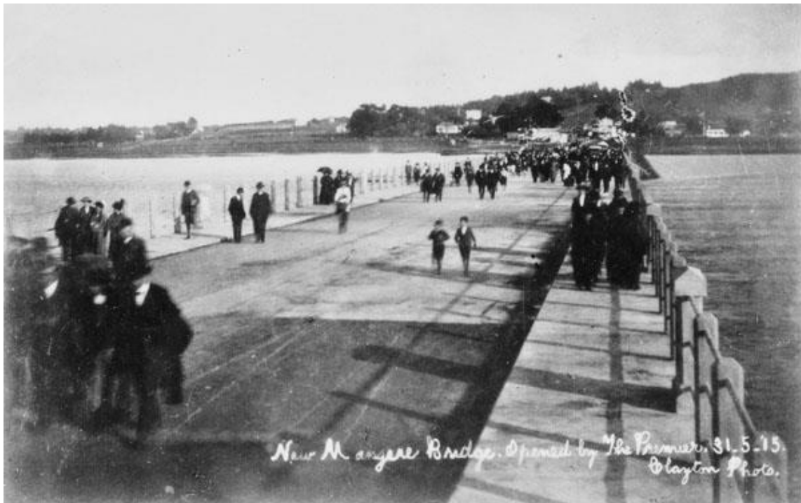
Figure 14: The scene after the opening of the second Māngere Bridge by Prime Minister William Ferguson Massey on 31 May 1915. Auckland Libraries Heritage Collections. Footprints 04404, photographer F Clayton.
