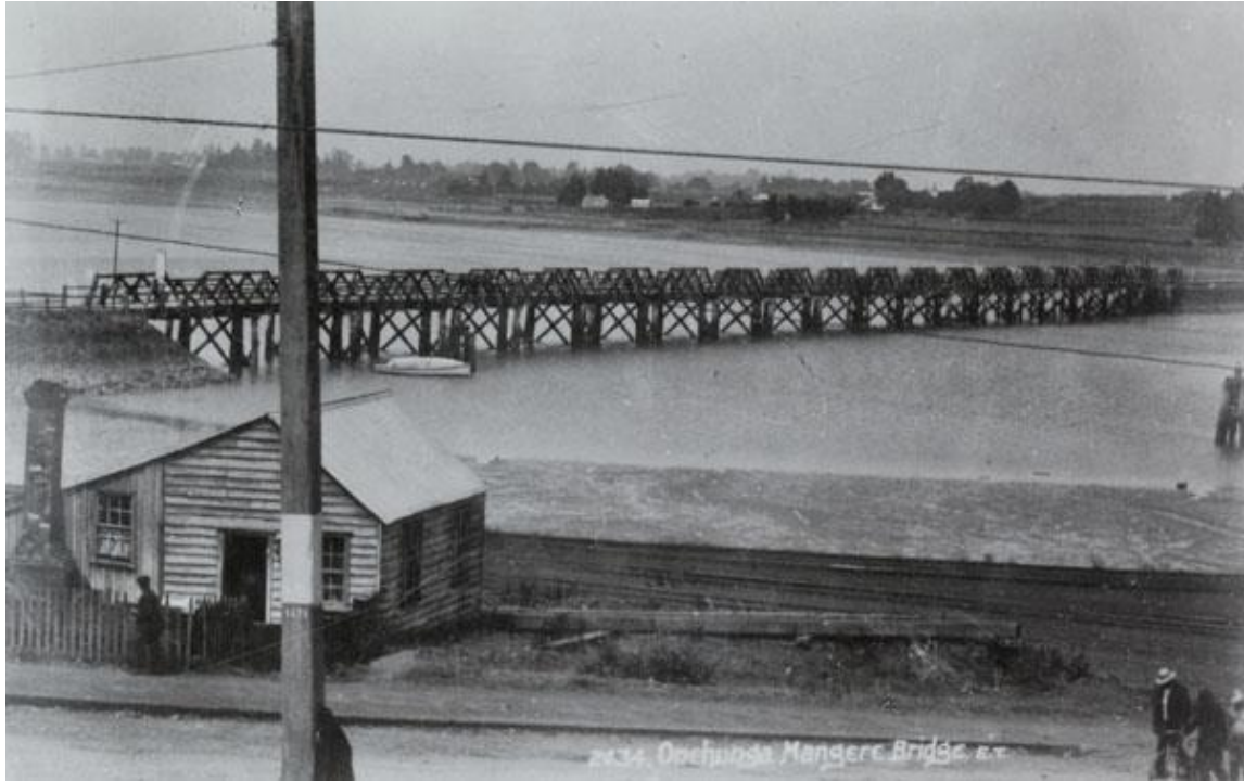
Figure 5: View of the first Māngere Bridge taken from the Onehunga side, c. 1907. Ernest Auckland Libraries Heritage Collections, Footprints 01120, photographer E De Tourret.
