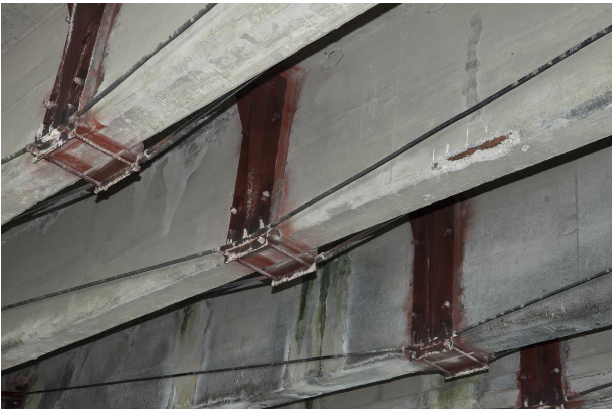
Figure 28:Bracket and tension wire repairs. Fraser Newman Photography
