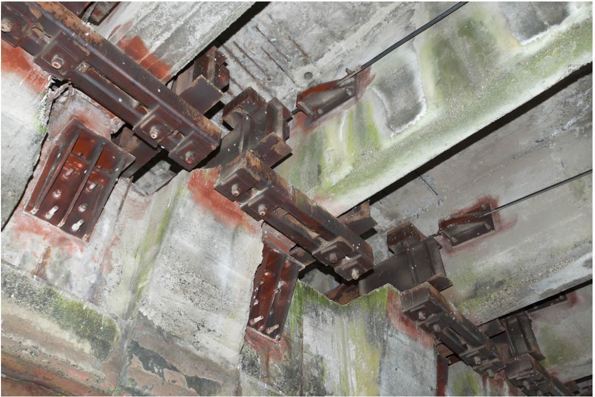
Figure 27:View of steel bracket repairs, date not confirmed. Fraser Newman Photography
