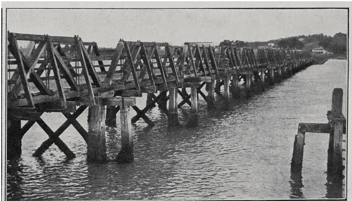
SHORTLY TO BE DEMOLISHED: THE BRIDGE CONNECTING MANGERE AND ONEHUNGA, WHICH IS TO BE REPLACED BY A MODERN STRUCTURE. P
