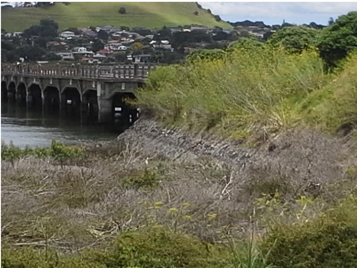
Figure 39: The east side of the northern embankment. Photo Matthew Felgate.
