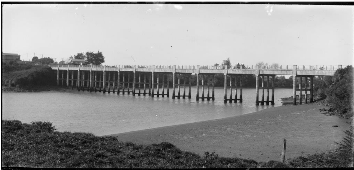
Figure 41: View towards the 1916 reinforced concrete Panmure Bridge 12 October 1927. Auckland Libraries Heritage Collections, 4-5866, photographer J D Richardson.
