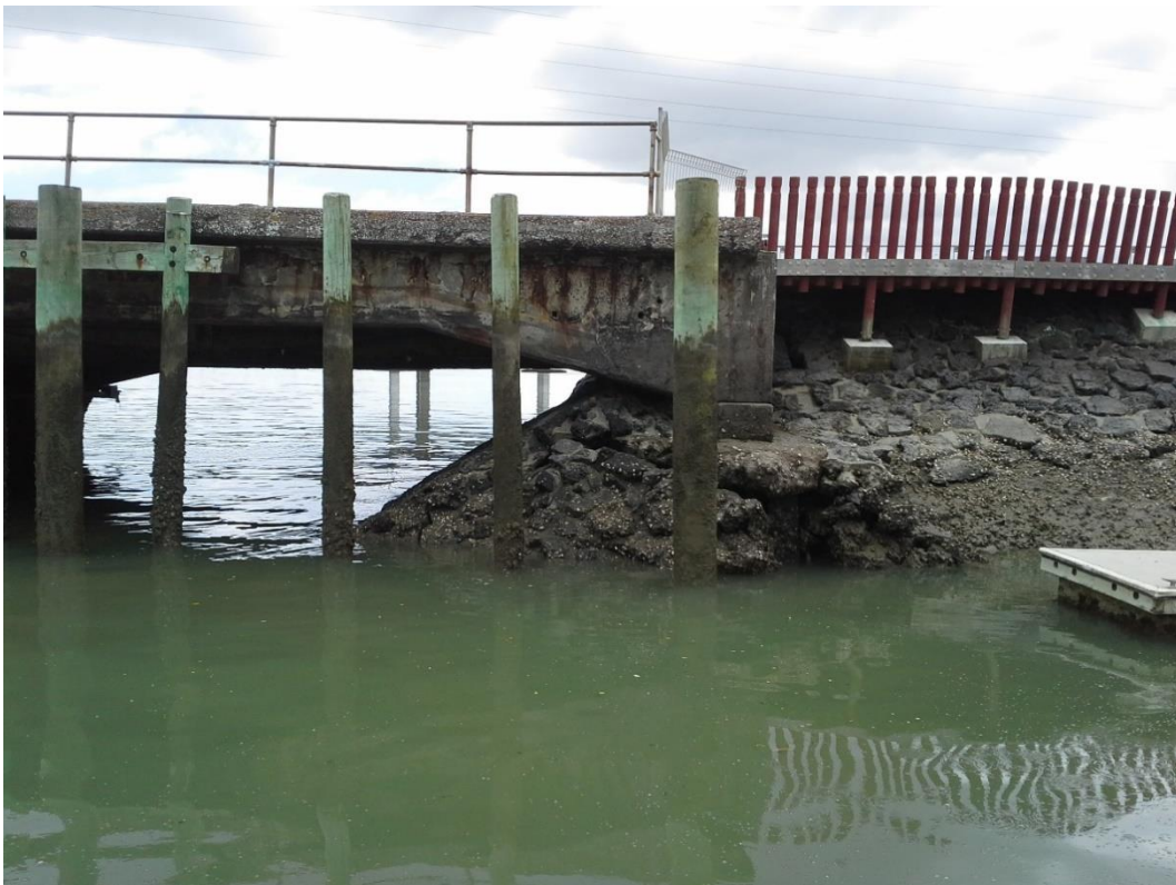
Figure 37: The southern abutment looking east. Photo Matthew Felgate.
