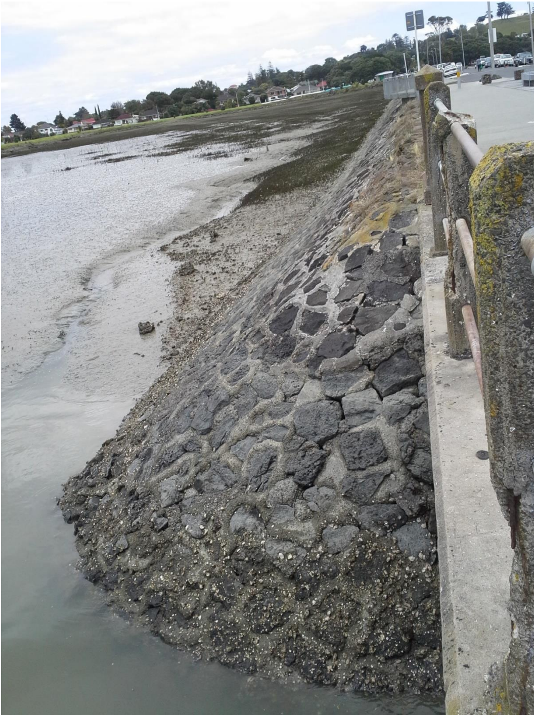
Figure 35: the eastern side of the southern abutment/causeway/embankment. Photo Matthew Felgate
