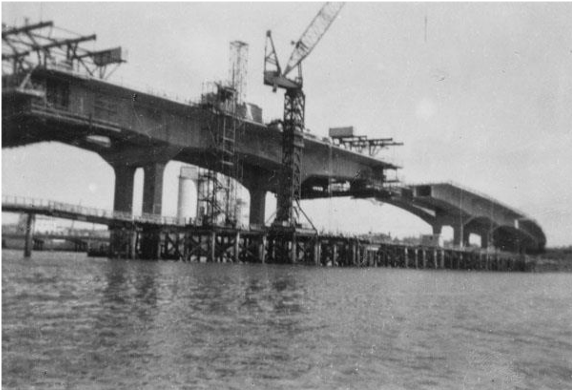
Figure 16: The third Māngere Bridge during construction, 1977. Auckland Libraries Heritage Collections, photographer unknown. Footprints 04411.
