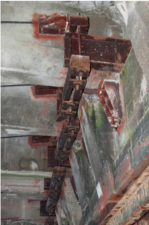
Figure 29: Repairs to support beams. Fraser Newman Photography
