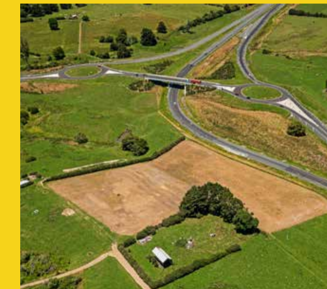
Partial 'half diamond' interchange, Waikato Expressway
