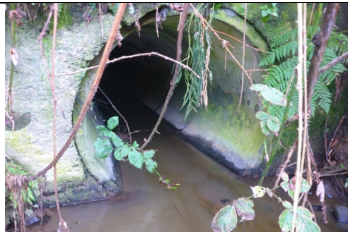
Stream 2 culvert beneath SH1 (12 April 2021)
