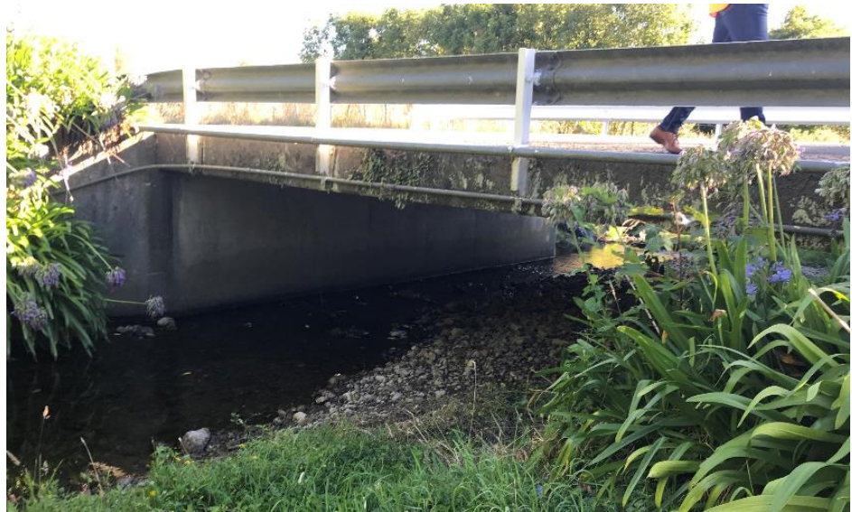
Figure F.27: Manakau Stream existing bridge downstream of proposed crossing
