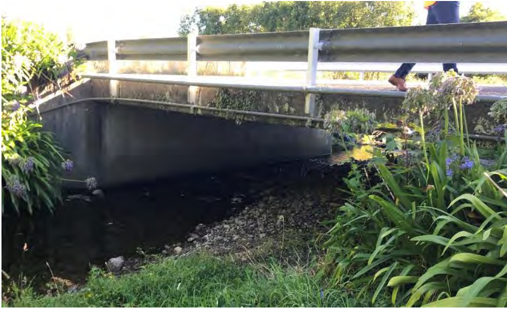
South_Manakau_rd DS Inside Bridge
