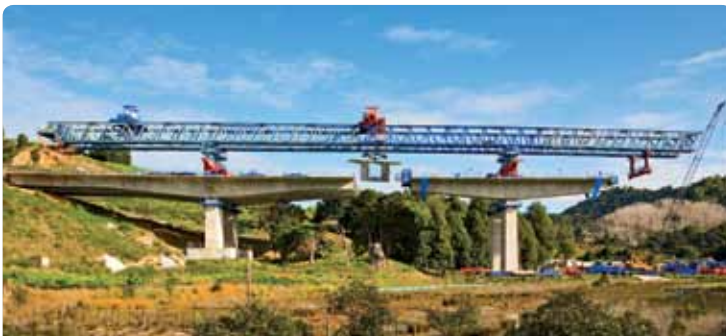
CITY SLICKER Having been used successfully to construct the bridge structures in the rural surrounds of the Northern Gateway Toll Rd, the 120-metre long Overhead Launching Gantry will undoubtedly provide an exciting new dimension to the Newmarket skyline.
