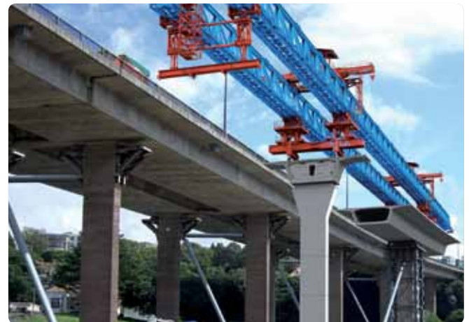
CITY SLICKER Having been used successfully to construct the bridge structures in the rural surrounds of the Northern Gateway Toll Rd, the 120-metre long Overhead Launching Gantry will undoubtedly provide an exciting new dimension to the Newmarket skyline.
