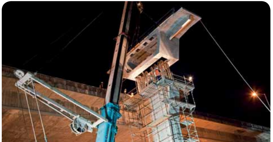
ONE UP ... 467 TO GO The first, 73-tonne bridge segment was lifted into place on the night of September 8. A further 42 segments will be installed by crane by the end of the year, to create a platform for the main construction equipment - a 700 tonne, 120 metre long Overhead Launching Gantry.
