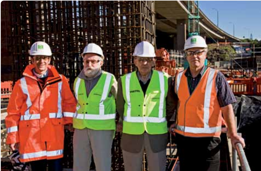
FROM GENERATION TO GENERATION Bryden McKinnell, Resident Engineer on the original viaduct project, and his Construction Manager, John Built, are flanked by the Newmarket Connection project's Construction Manager and Project Manager, Patrick Arnold and Ian Harbeck (l-r).
