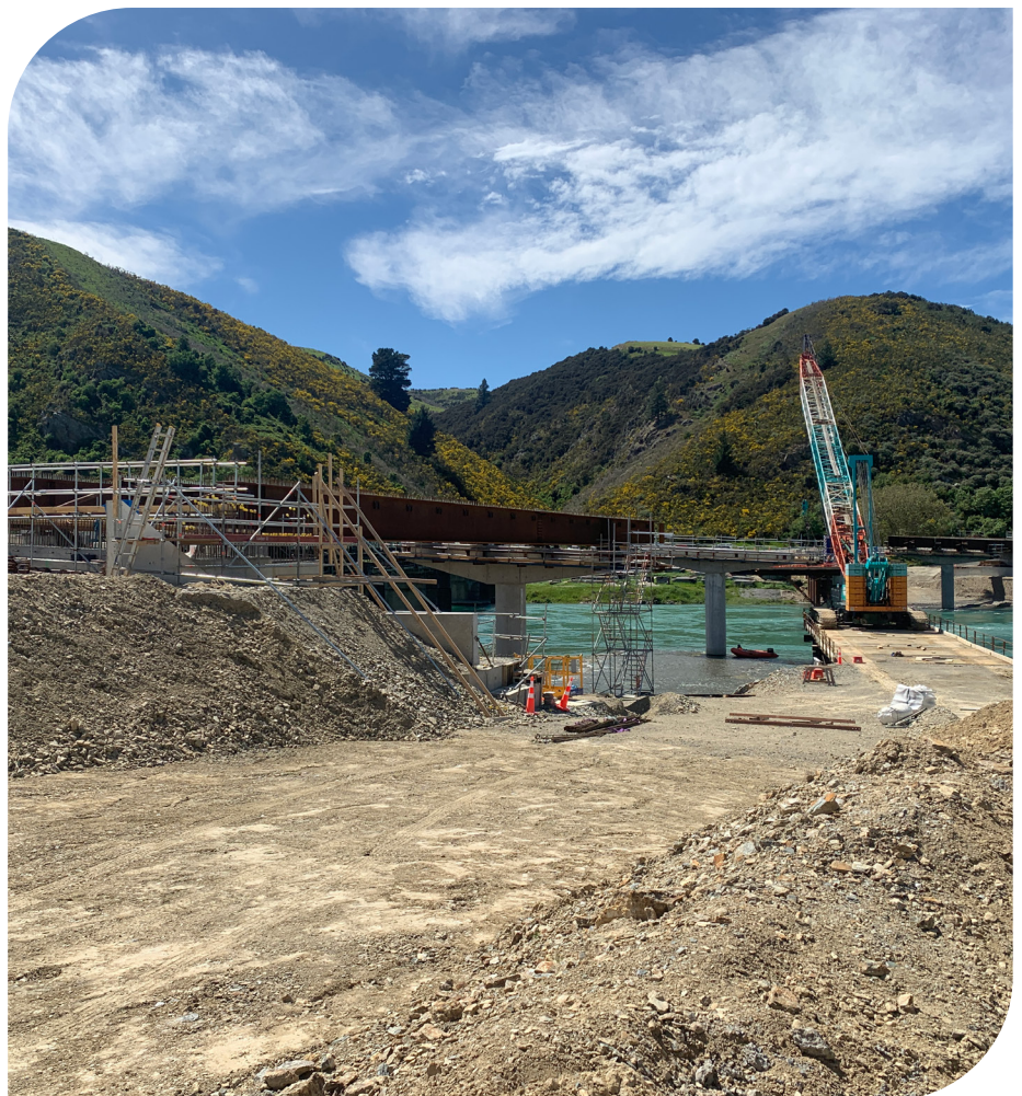
The new bridge western abutment looking toward the eastern bank
