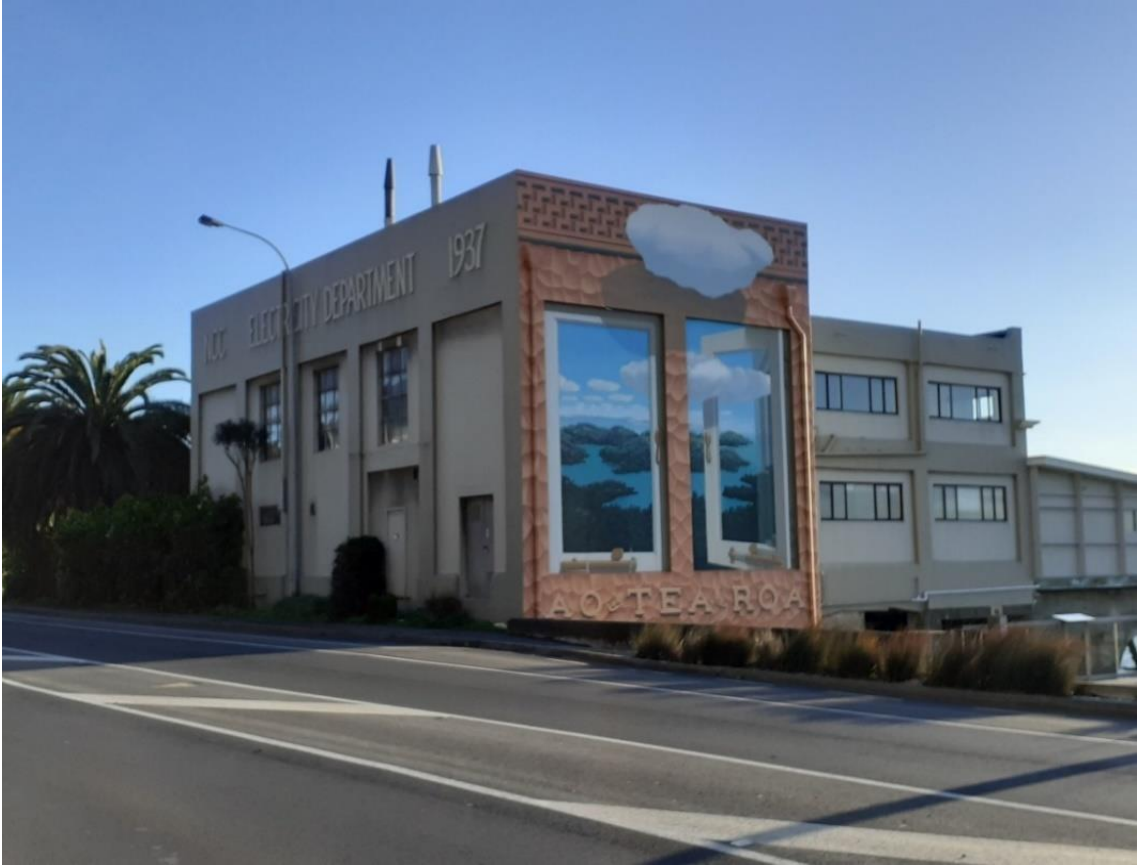
Figure 16 : Photo of Street Frontage of Powerhouse
