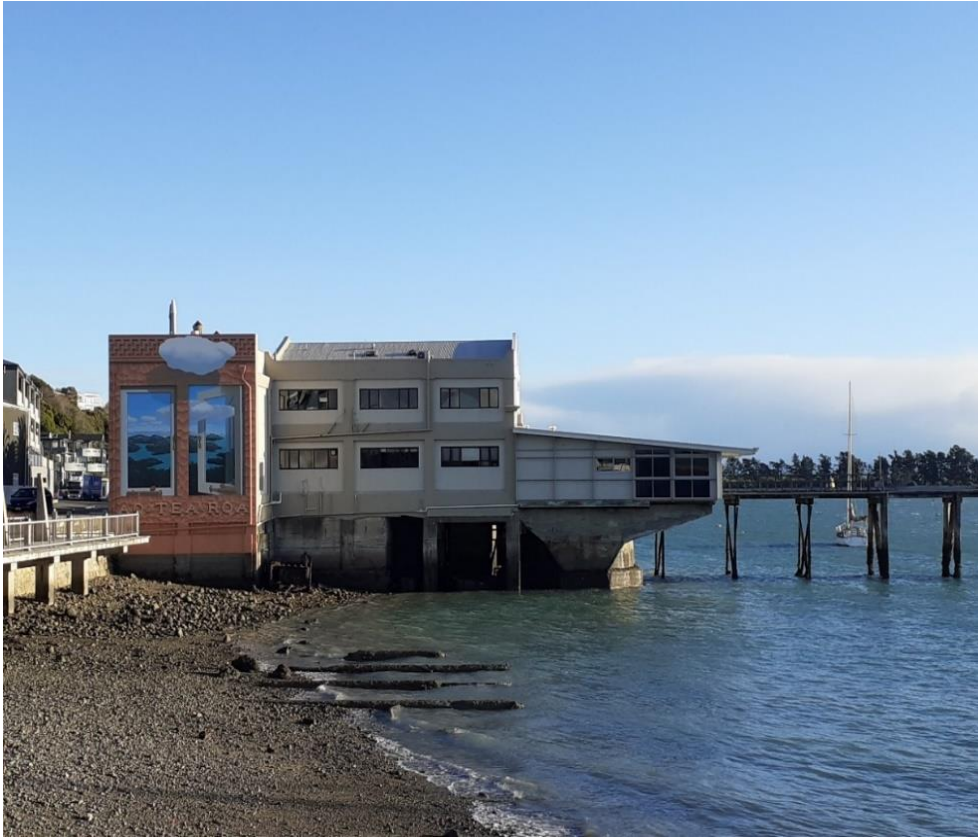
Figure 17 : Powerhouse northern elevation
