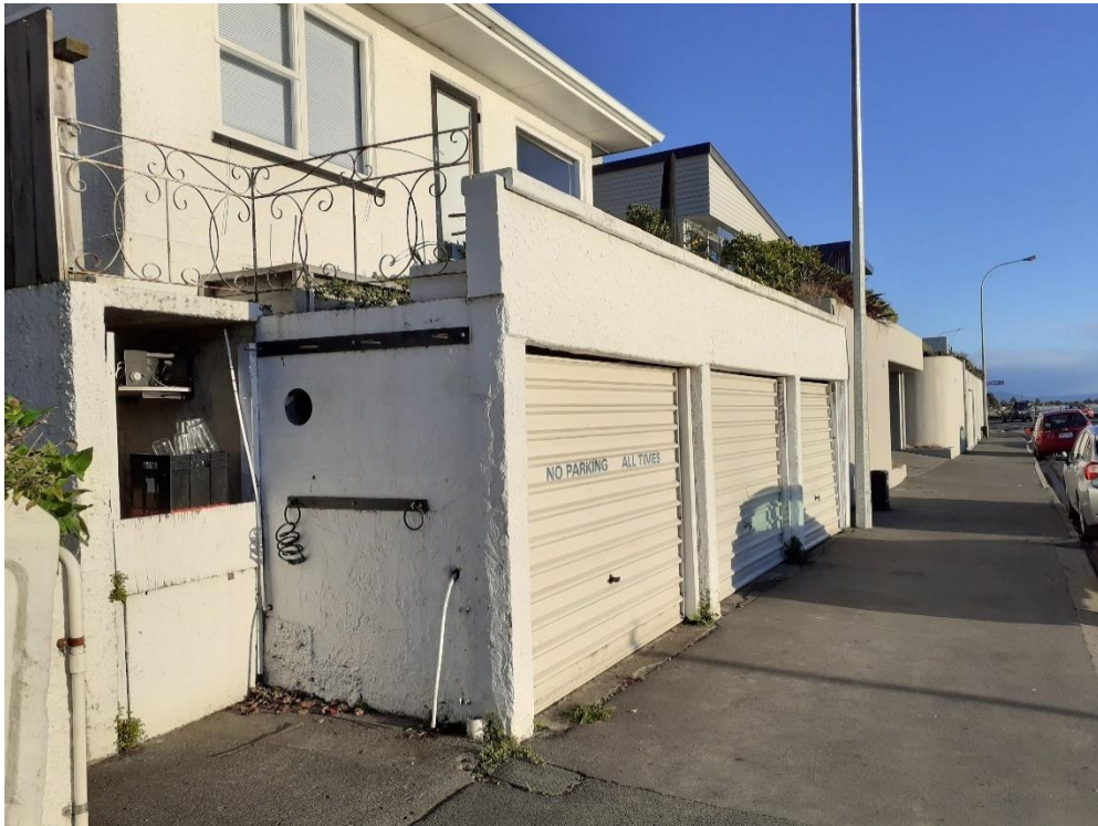
Figure 8 : Photo of 351 Wakefield Quay (restaurant storage/office space)
