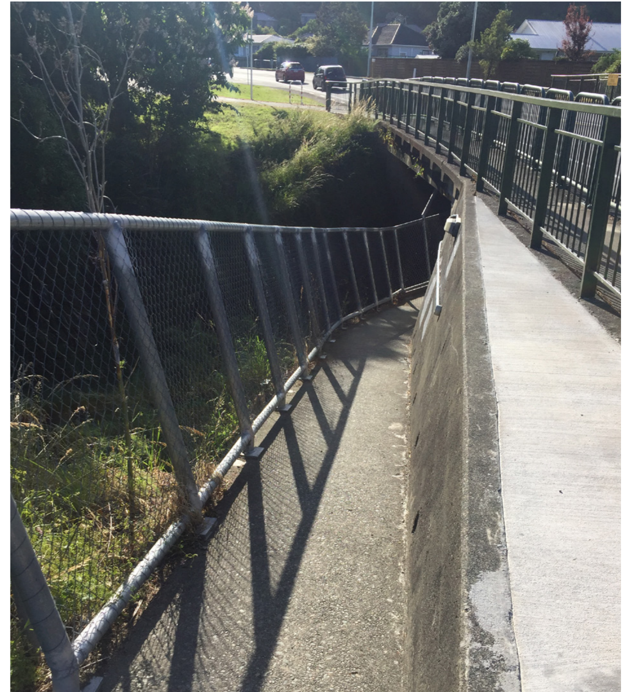
Figure 14: Jenkins Creek Underpass
