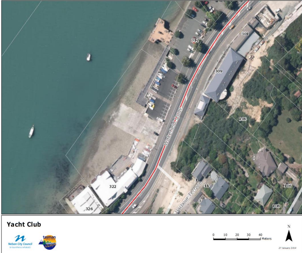
Figure 11 : Aerial of the Nelson Yacht Club site
