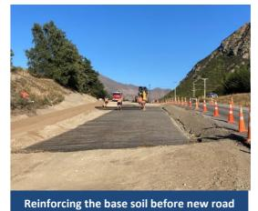
Reinforcing the base soil before new road construction starts on inbound Luggate leg
