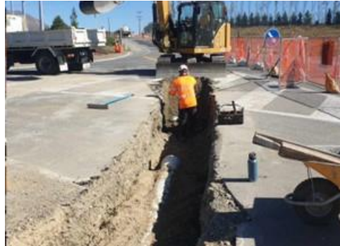
Trenching at Ballantyne Road, getting ready to install upgraded underground services.
