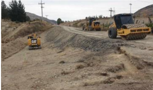
Earthworks along Riverbank Road south to support widening the road.
