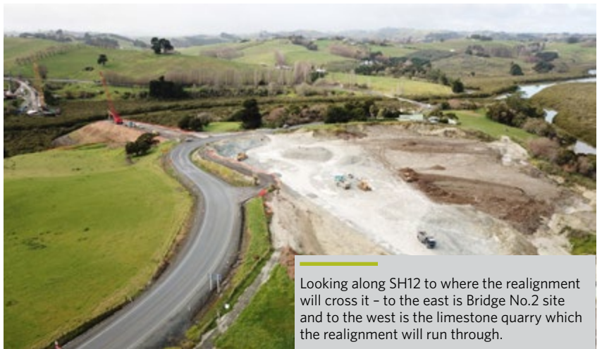
Earthworks at the western end of the realignment involve cutting down the paddocks and then materials, including limestone from the local quarry to form part of the subgrade, are built up in layers to construct the new road carriageway.
