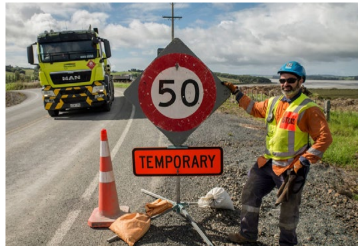
STMS Owen Vercoe carrying out a site check.
