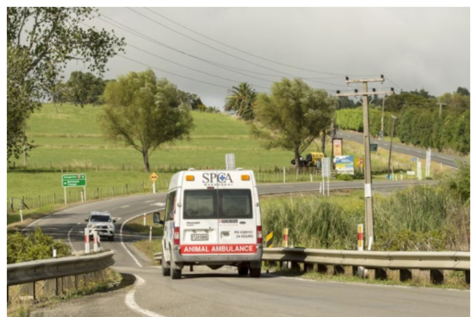
Hardies Bridge is one of Matakohe's two, single lane bridges that is being retired from the state highway network.
