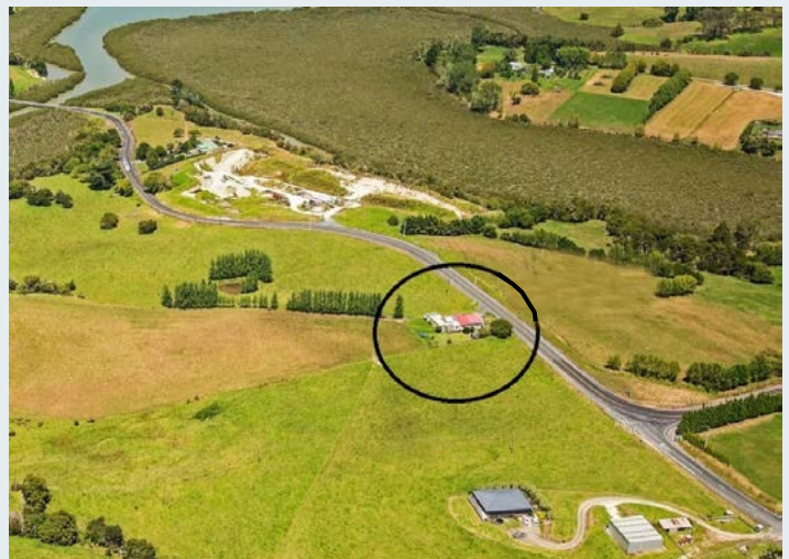
The property that will become the site office and compound
