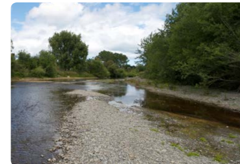
THE FORM OF THE RIP RAP AROUND THE BRIDGE COLUMNS SHALL RESEMBLE THE NATURAL BRAIDED RIVER ISLANDS FOUND NATURALLY IN WATERCOURSES IN THE REGION
