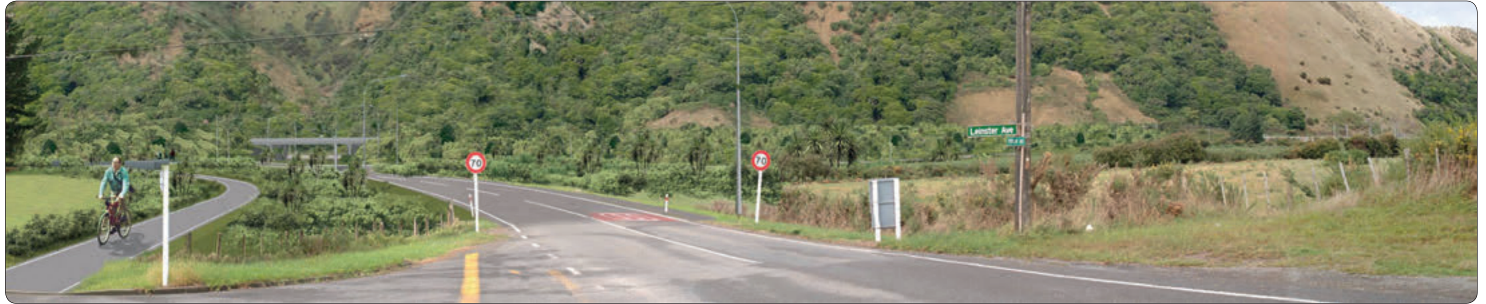
AEE VISUALISATION - POPLAR AVENUE CROSSING (NORTH SIDE OF POPLAR LOOKING EAST) SITUATION FOLLOWING CONSTRUCTION
