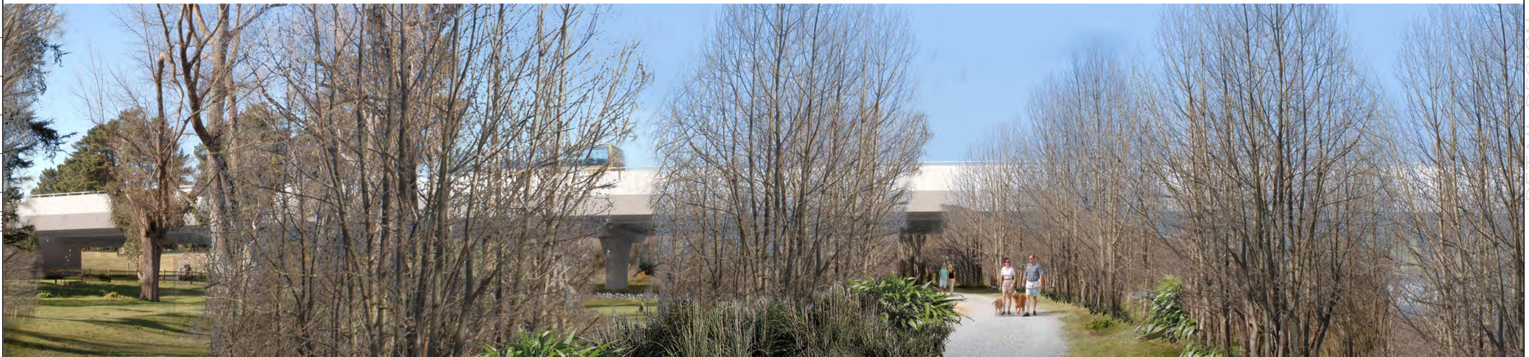
WITH MITIGATION PLANTING AT APPROXIMATELY 10 YEARS
