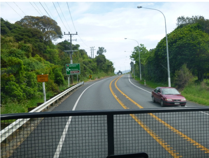
Figure 8: Southbound approach showing guide sign
