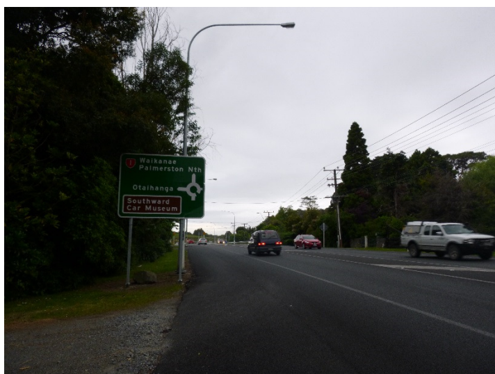
Figure 4: Northbound approach to the roundabout, showing the existing guide sign
