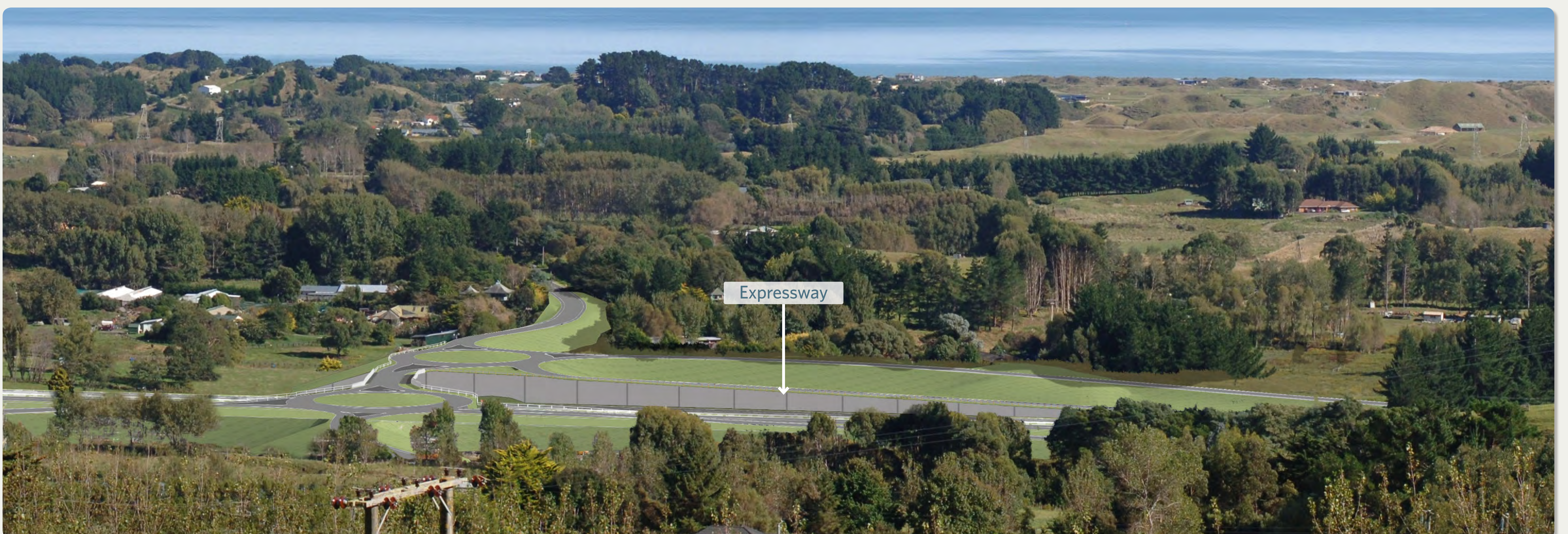
Indicative view of expressway from Hadfield Road area looking west - before mitigation work.
