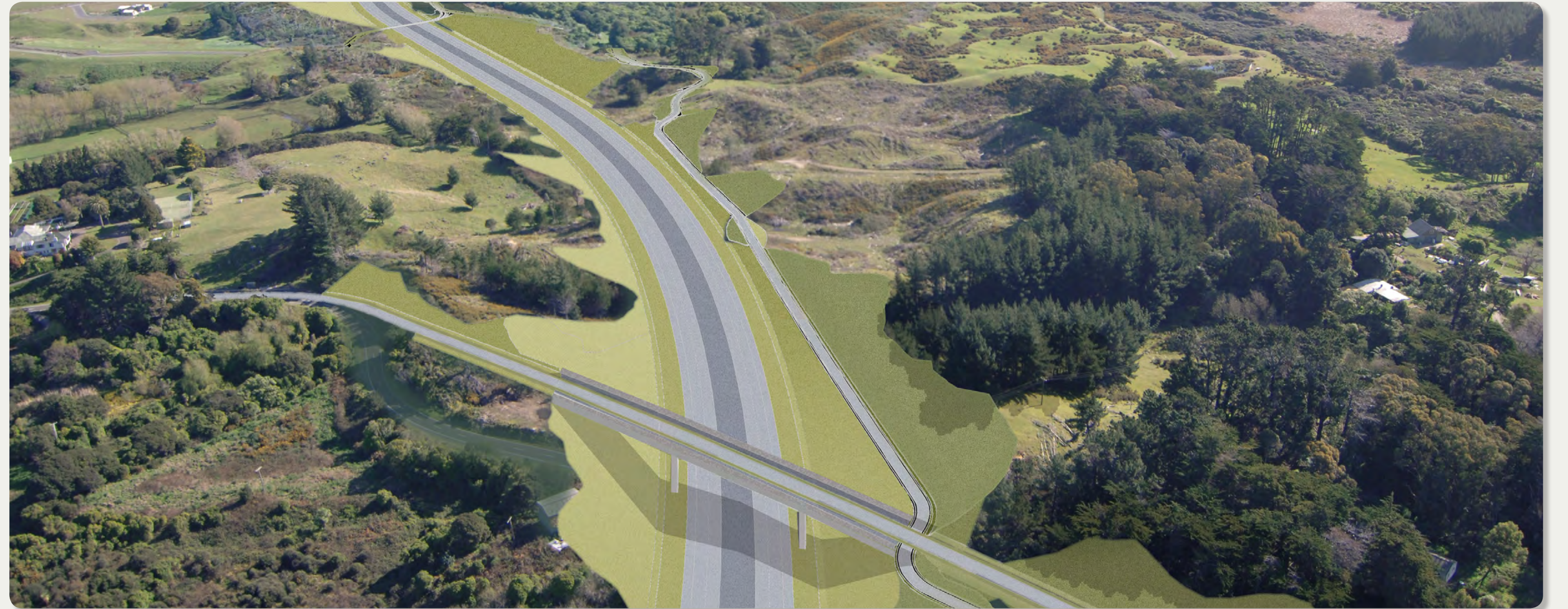
Indicative aerial view of the Ngarara Road expressway overbridge looking south. The shared cycle/walk path can be seen on the west (right) side - before mitigation work.
