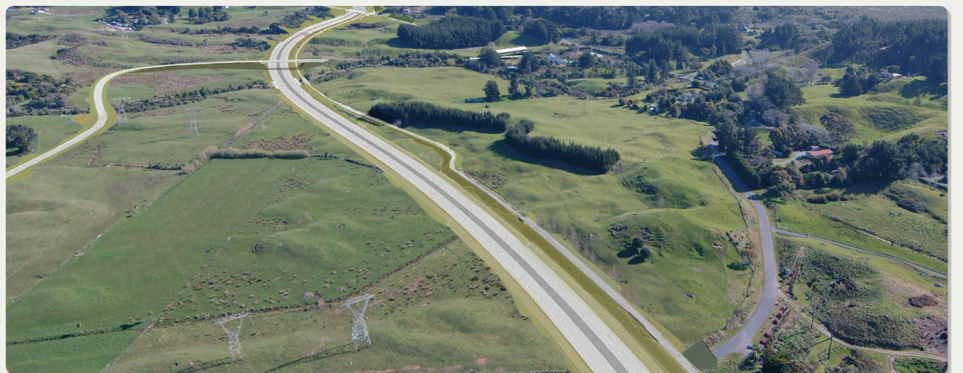
Indicative aerial view of the new connection overbridge looking south. Smithfield Road is closed – access to Nga Manu (in the top left corner of the image) will be from the new local road. The shared cycle/walk path can be seen on the west (right) side - before mitigation work.
