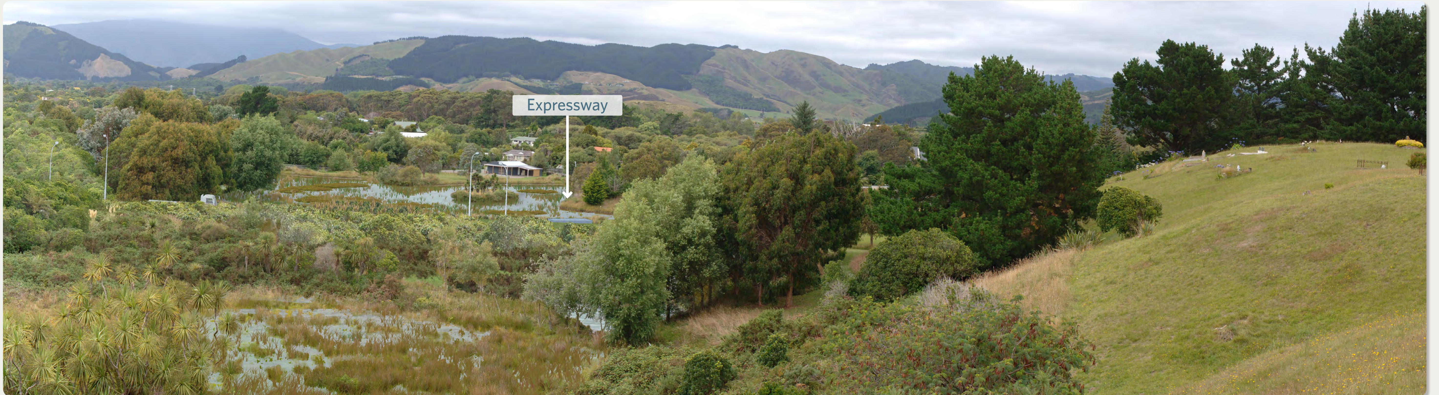
The mitigation treatment includes the natural shaping of landforms and replanting with dense native planting. Noise barriers - bunds and walls - will also be incorporated in some areas with their design to respond to the adjacent property. The wetland areas will be extended and enhanced, and will have a stormwater management function.
