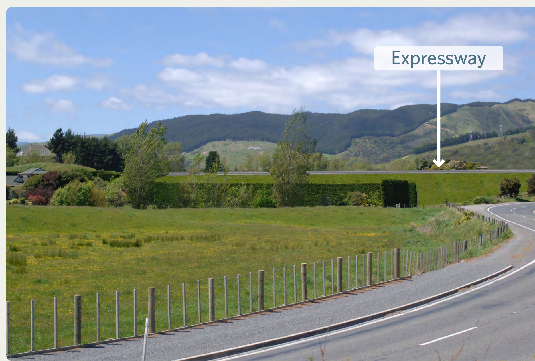
Indicative street level view looking east on Otaihanga Road - before mitigation work.
