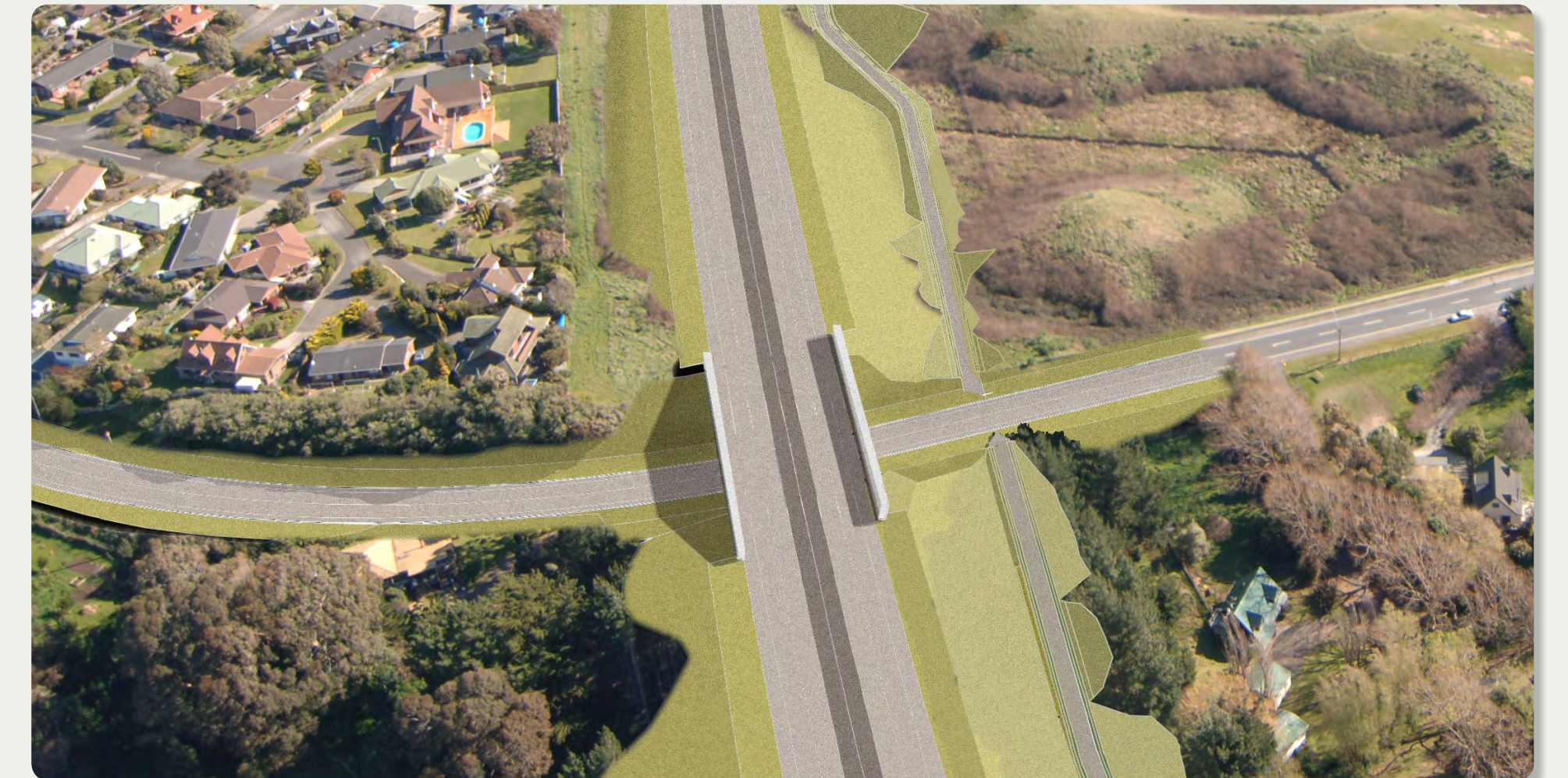
Indicative aerial view of the Mazengarb Road expressway bridge. The shared cycle/walk path can be seen on the right side - before mitigation work.
