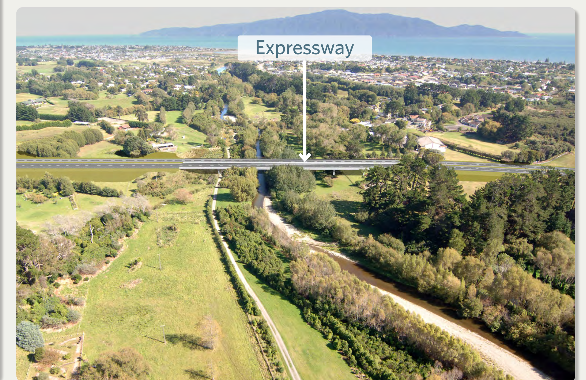
Indicative aerial view of the Waikanae River expressway bridge - before mitigation work.
