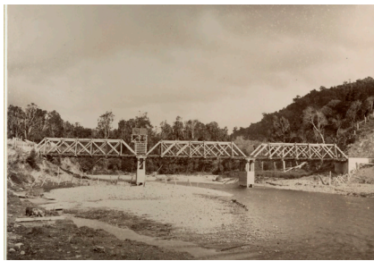
Wellington and Manawatu Railway bridge over Waikanae river. Levin, William Hort, 1845-1893.
