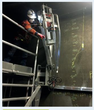
The working platform and drill rig designed for ensuring tunnel duct panels loading restrictions and increased hole drilling efficiencies are achieved during the installation of 9km of new pipe, held in place by 1326 brackets.
