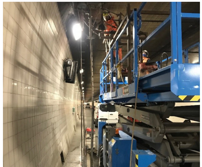
Teams installing the new fire protection pipework inside the tunnel.
