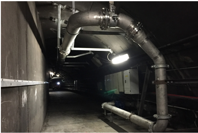
New wastewater pipeline suspended from the duct ceiling.
