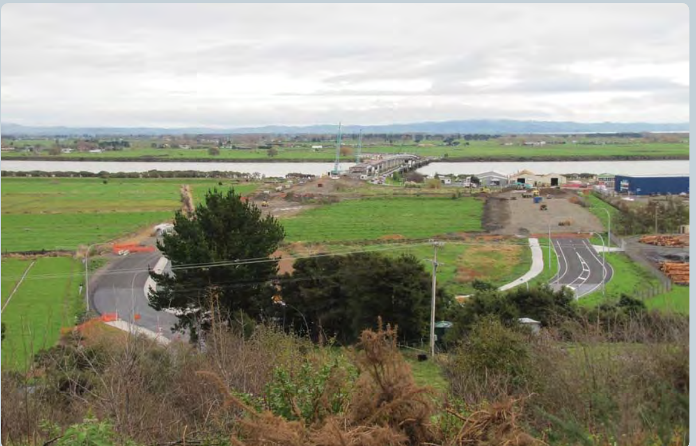
The SH25/26 roundabout is obscured by the trees in the foreground. The road on the left shows the route the approach roads will take. The road on the right will connect with a future local link road from the roundabout to the Kopu industrial area
