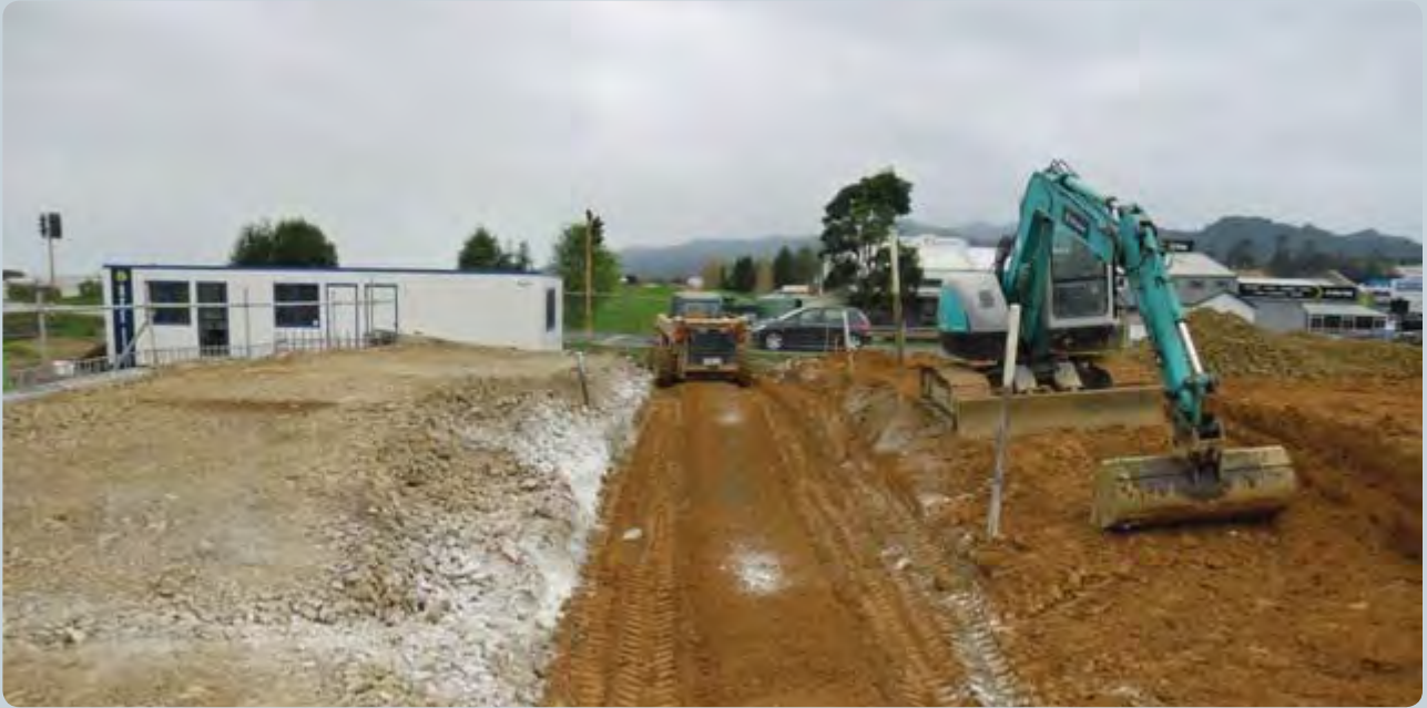
To build the western approach to the bridge, a gap was dug in the Waihou River stopbank. Construction staff are shown replacing the stopbank materials prior to building the approach road
