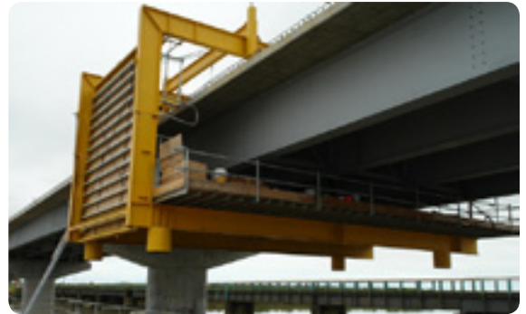
The platform for the removal of concrete formwork
